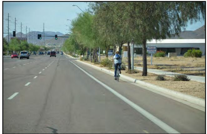
Bike lanes exist between SR-101 and Happy Valley Road (looking northbound)
