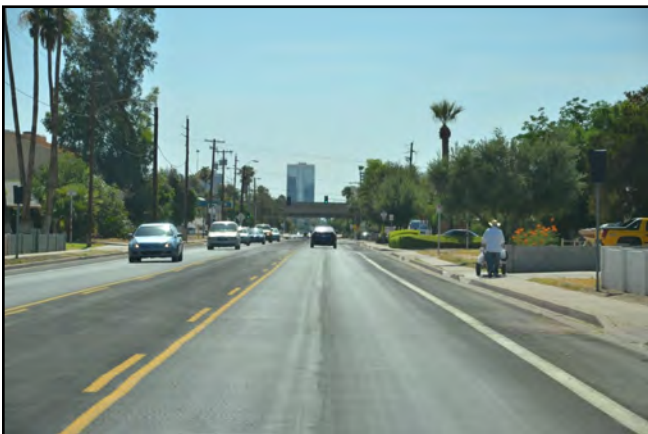
Looking west on Osborn Road approaching SR-51
