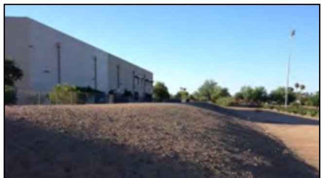
47th Avenue and Sweetwater Avenue berm - north end
