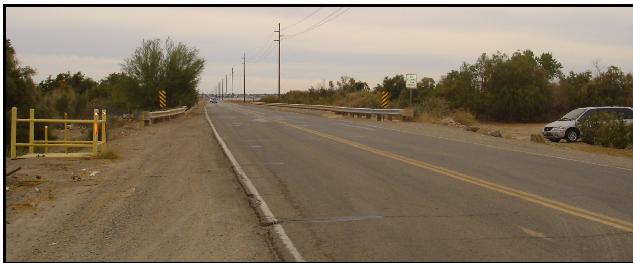
Figure 11: Bridge on Laguna Dam Road
