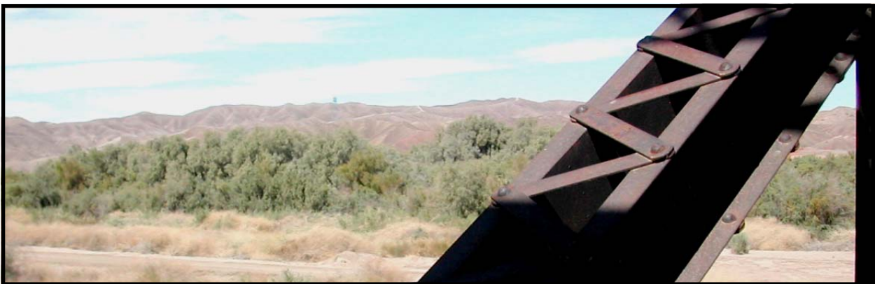
Figure 33: Gila River & the McPhaul Bridge
