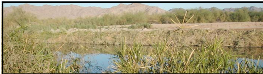
Figure 1: Gila Gravity Main Canal
