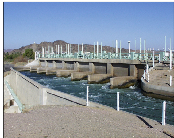
Figure 18: Gila Gravity Canal Headworks 4
