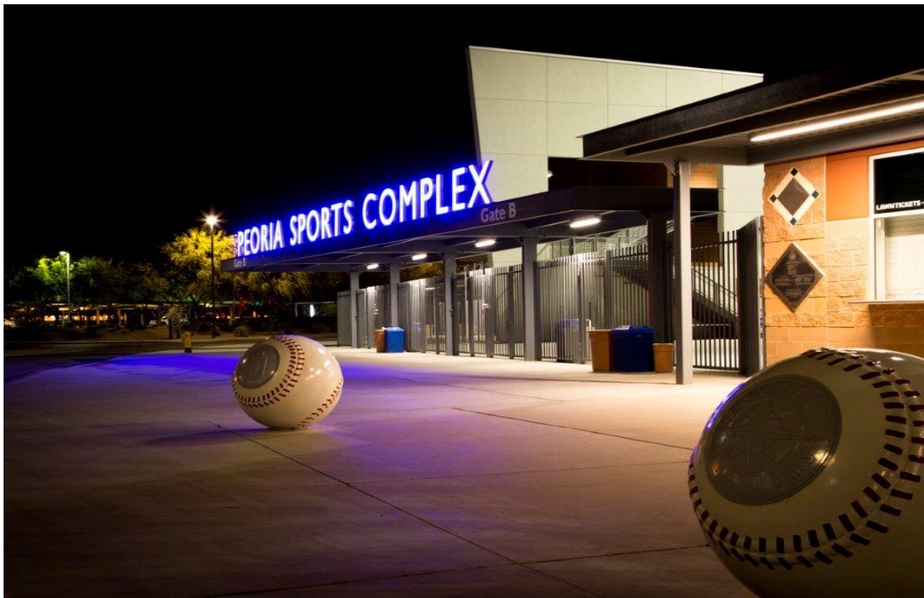
The front entrance of the Peoria Sports Complex was recently renovated as part of the city's Capital Improvement Plan.
