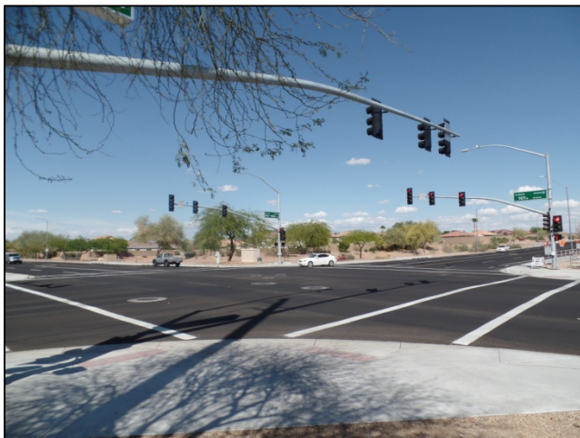
Deer Valley Road Improvements
