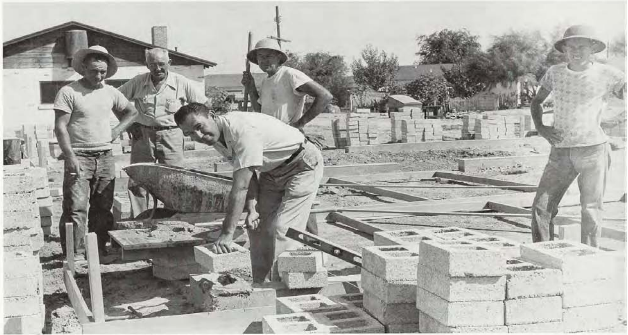
Volunteers look on as Mayor William Killip lays the southwest corner brick for the first Town Hall and fire Station in 1948. The Boy Scout Lodge appears in the background. Pictured above left to right: Farris (Bing) Crosley (building contractor), Ben Veneklassen (Town Clerk), Chick Viehl (citizen), Mayor William Killip and Ronnie Loutzenheiser (citizen).
