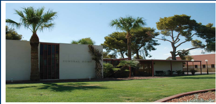
Thompson's West Funeral Chapel Before Renovations
