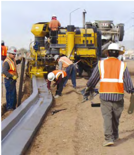
Curb Gutters Installed
