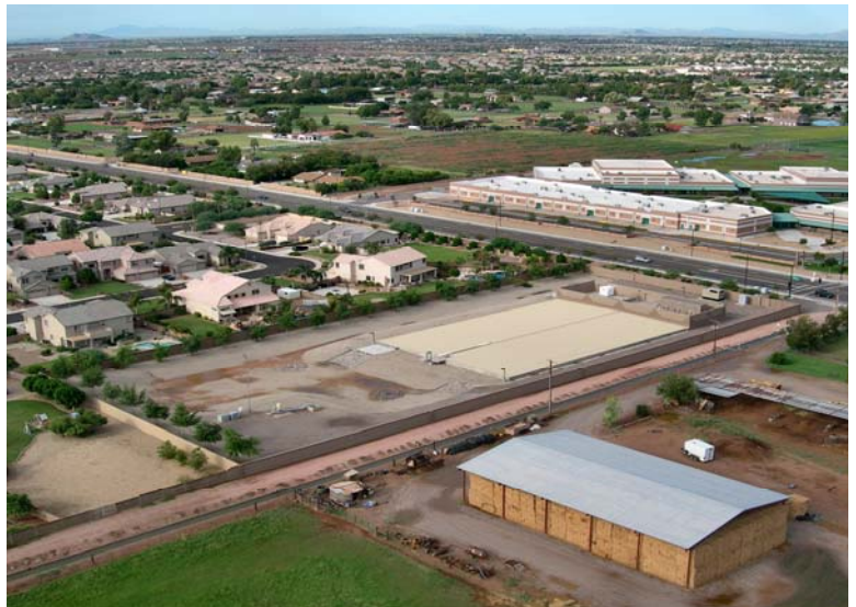
4 Million Gallon (MG) Reservoir - Lindsay Road
