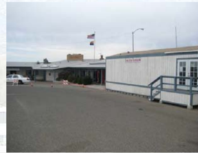
Terminal Building (Exterior)
