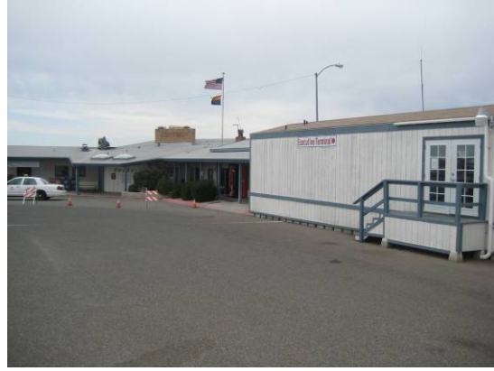
Terminal Building (Exterior)
