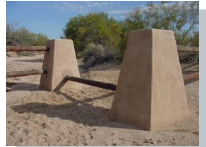
Constructed barriers prohibit off road vehicles use in the Desert Foothills Area
