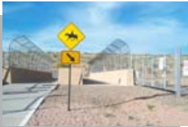
A bridge over the Central Arizona Project Canal provides a major trail connection.
