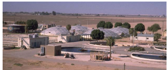
Existing Water Pollution Control Facility
