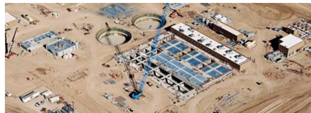
New East Mesa Water Pollution Control Facility
