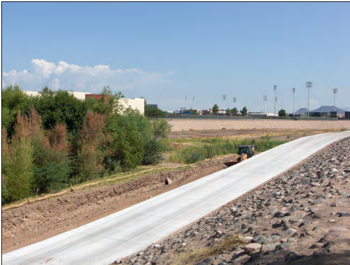
Construction is nearly complete on the New River Trail system.
