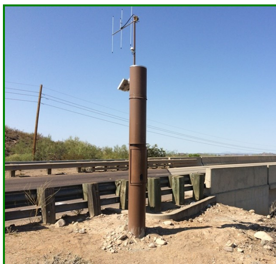
Skunk Creek at Carefree Highway Installed August 18, 2015
