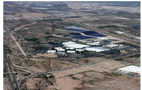
UA Tech Park, looking northwest.
