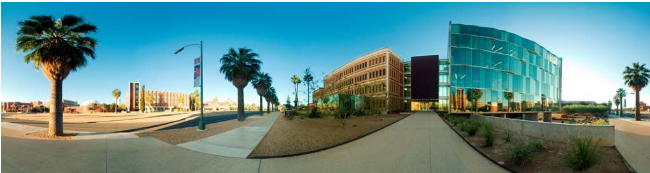
Optical Sciences building on the UA main mall.
