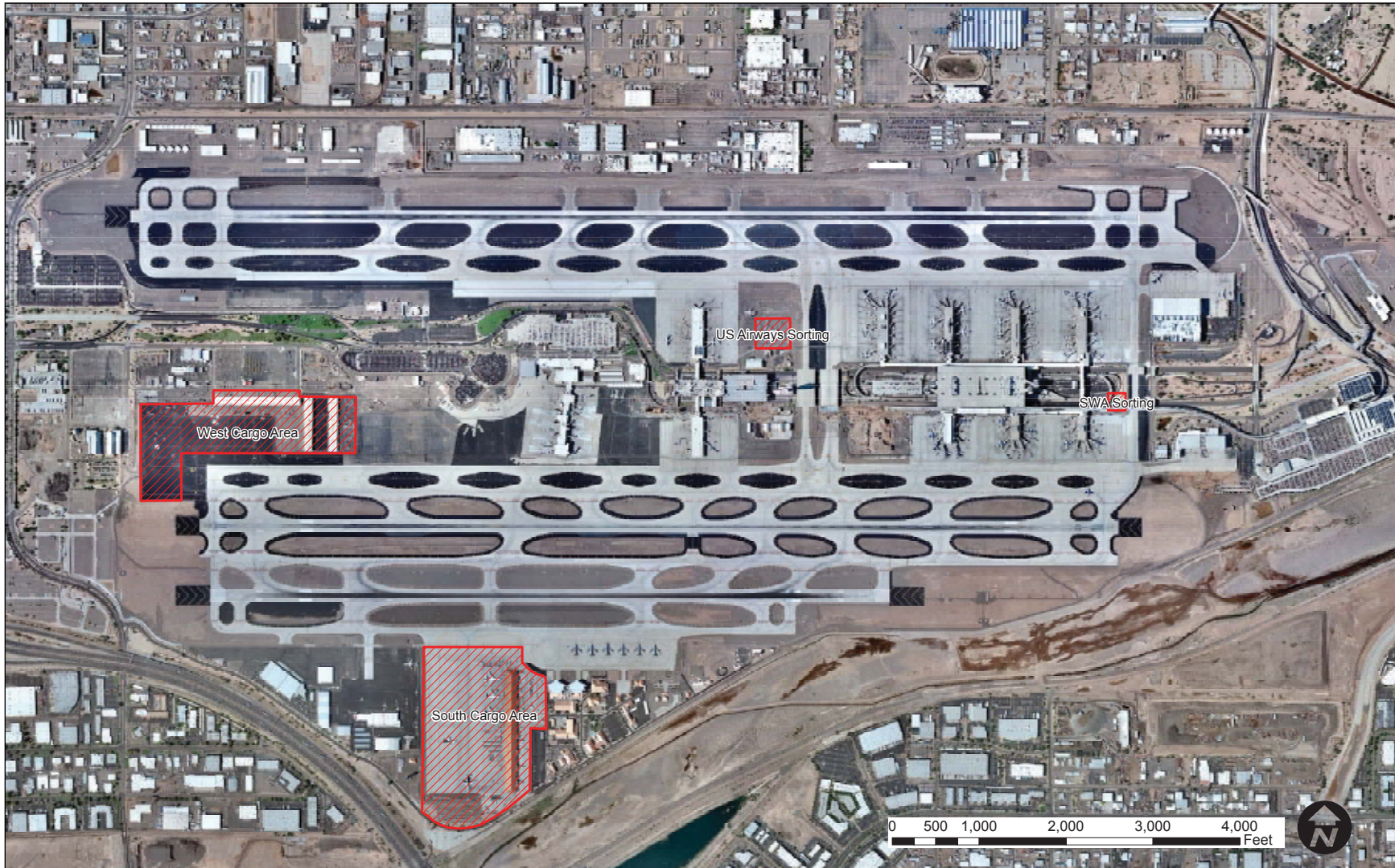
Exhibit 5.1: Phoenix Sky Harbor International Airport - Cargo Area
