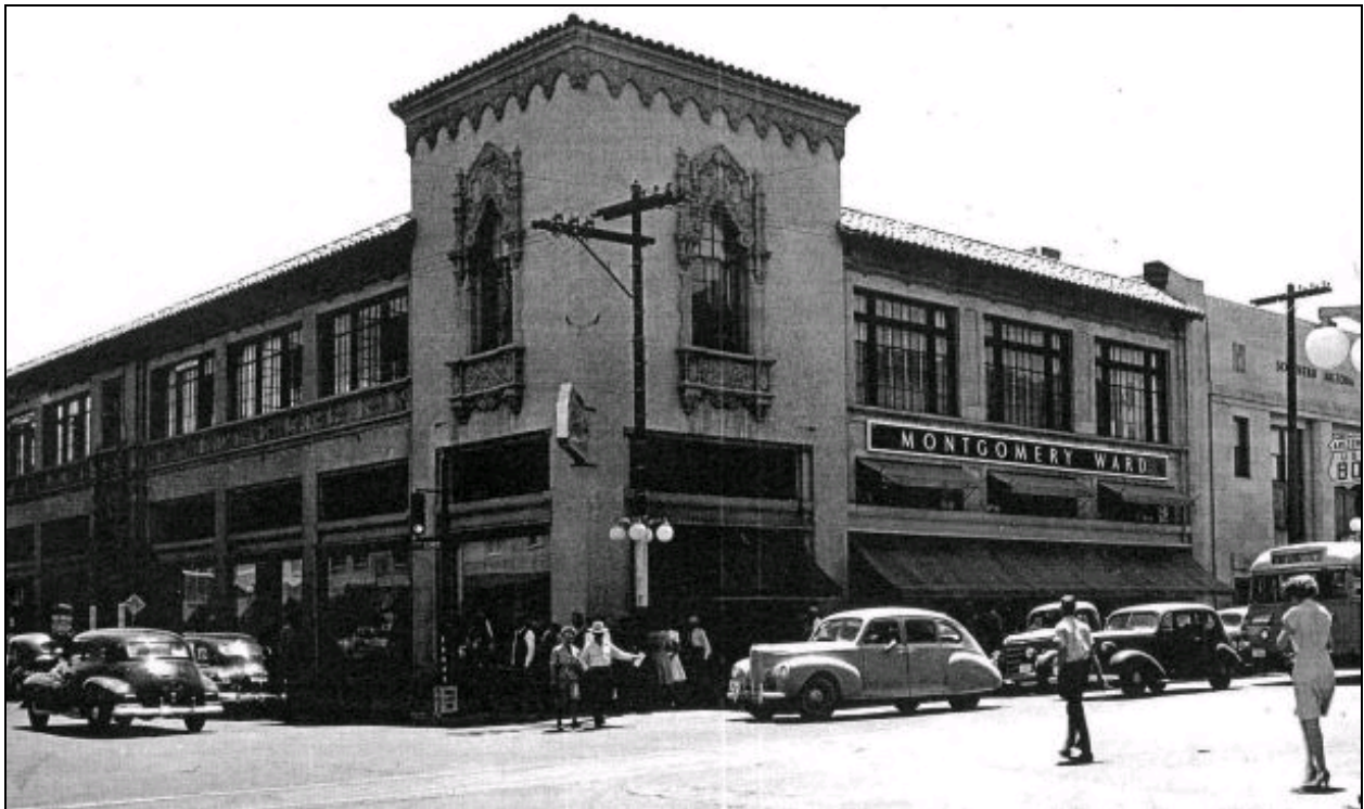
Undated photograph of the historic Roy Place Building in Tucson.
