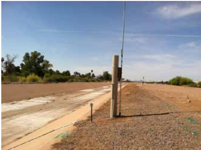
EMF below Powerline Floodway, #6758
