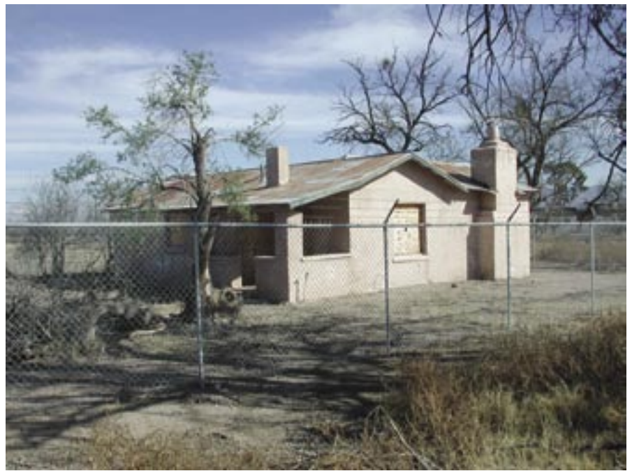
View looking northeast from the southwest Photo courtesy of Poster Frost Associates, 2004
