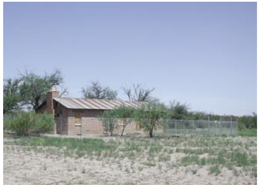
View looking northwest from the southeast Photo courtesy of Poster Frost Associates, 2004
