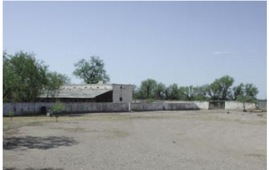
View looking southeast from the northwest Photo courtesy of Poster Frost Associates, 2004
