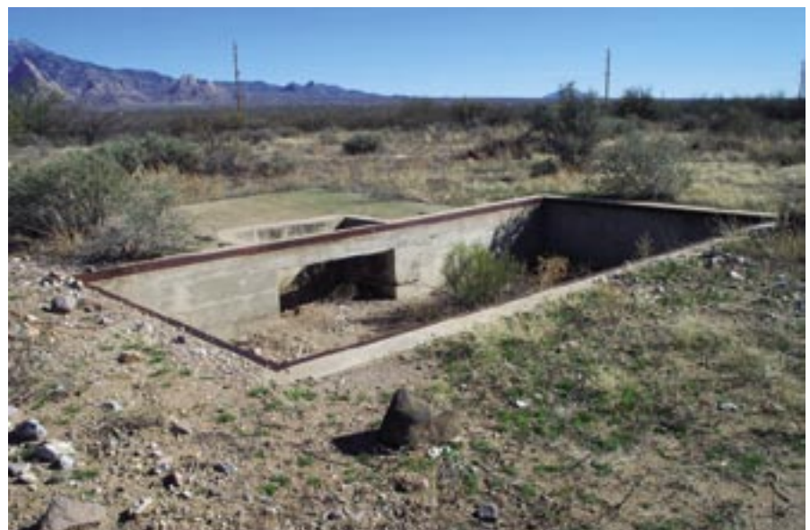
Truck scale foundation associated with AZ DD:4:48
