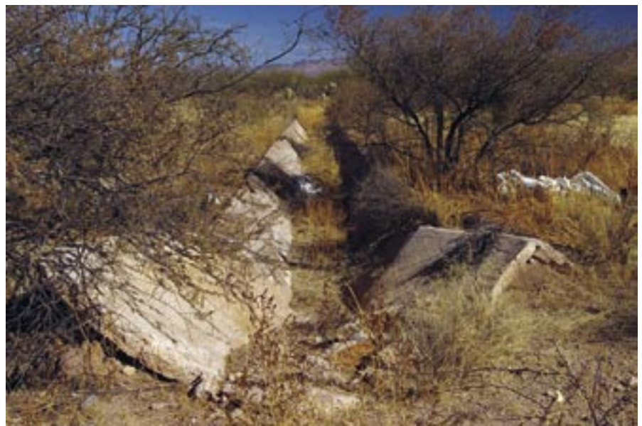
Typical concrete lined irrigation ditch
