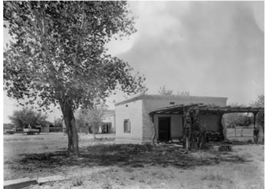
View from the northeast looking southwest, before addition Photo courtesy of Diana Hadley, date unknown
