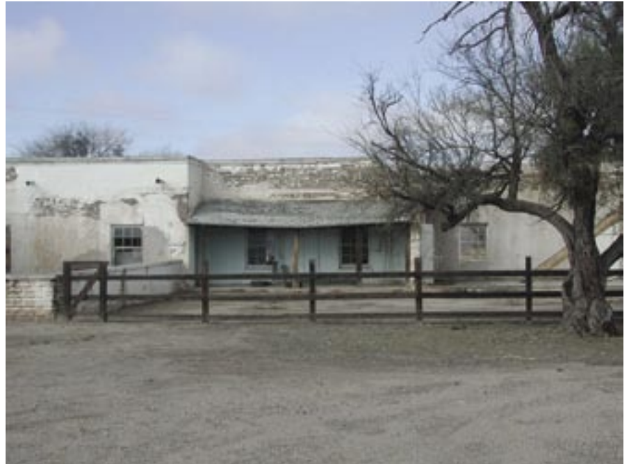
View looking west from the east Photo courtesy of Poster Frost Associates, 2004
