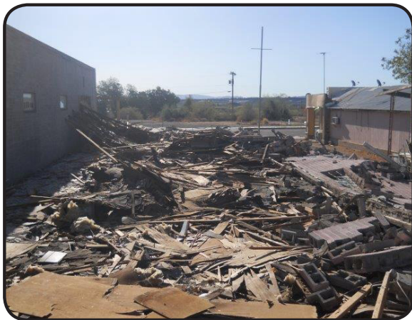
Brownfields and Demolition Project in Ajo, Arizona
