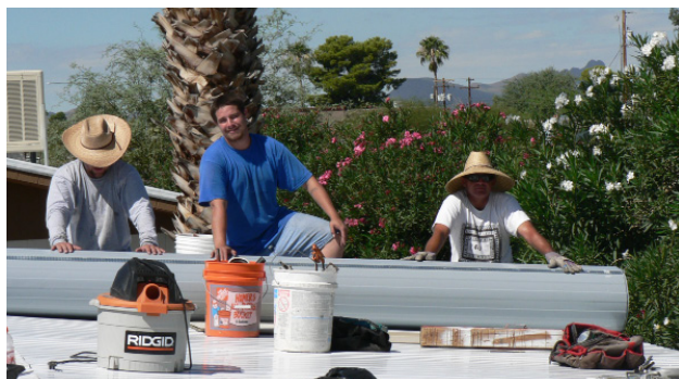
Program contractors weatherize a participant's home.
