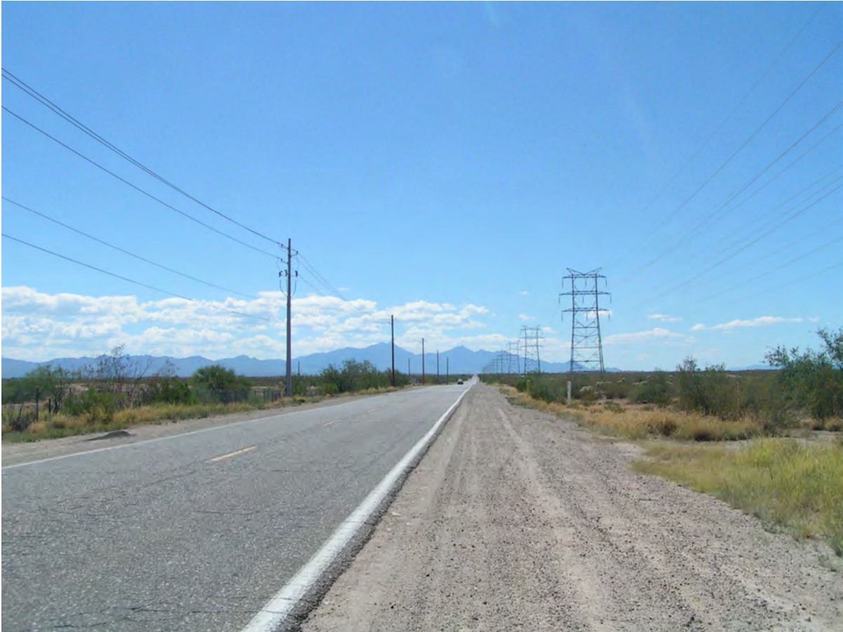
View of Swan Road, south of Los Reales Road, looking south. This views shows the 138,000 power lines on the west side of the road, and the 14,000 volt power lines on the east side of the road
