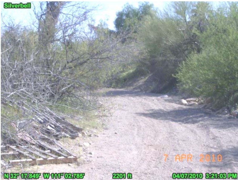
Figure 5.1. Del Cerro Wash Photo 1. The center of the flow path of the Del Cerro Wash immediately upstream of Silverbell Rd.
