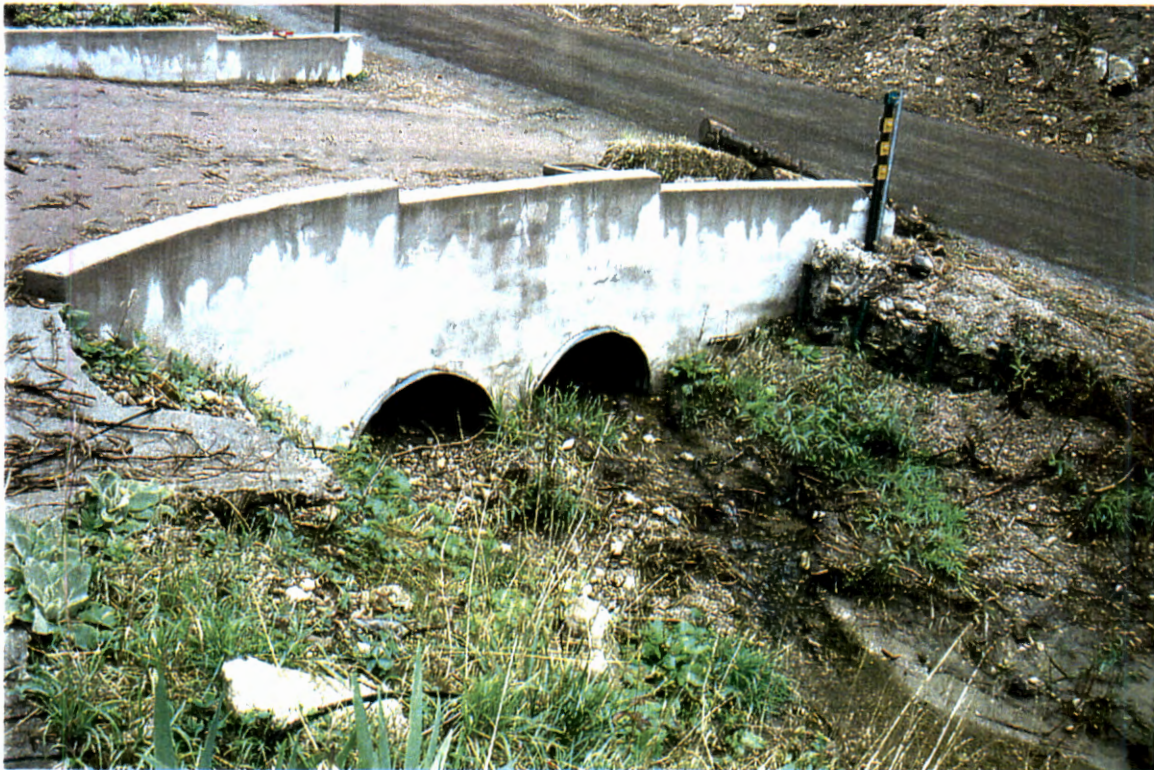
Picture 106. Downstream of driveway culvert looking upstream at 2-36" CMPs (# 19).
