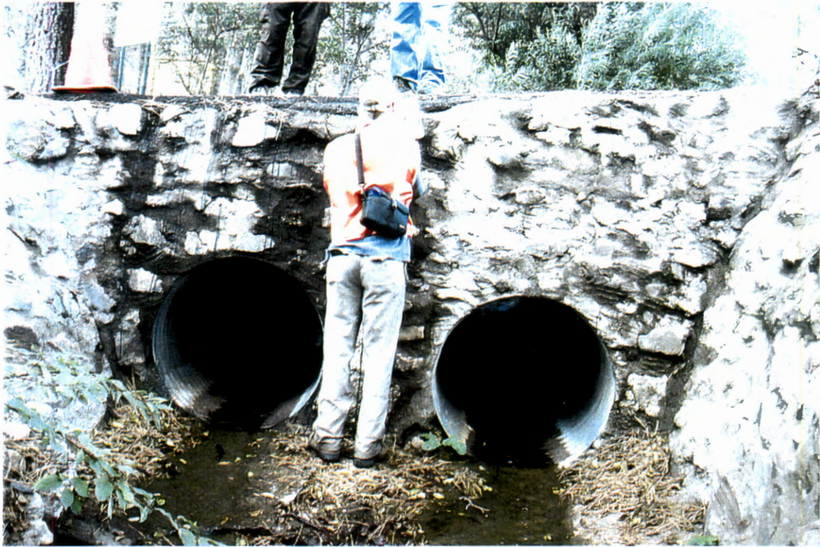
Picture 55. Centerline of channel looking upstream at 2-36" CMPs (# 6).
