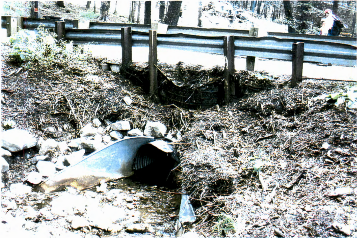
Picture 47. Upstream of Goat Hill Road culvert looking downstream at culvert (# 4).
