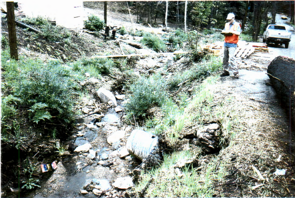
Picture 79. Downstream of culvert (# 13) looking downstream at centerline of channel.
