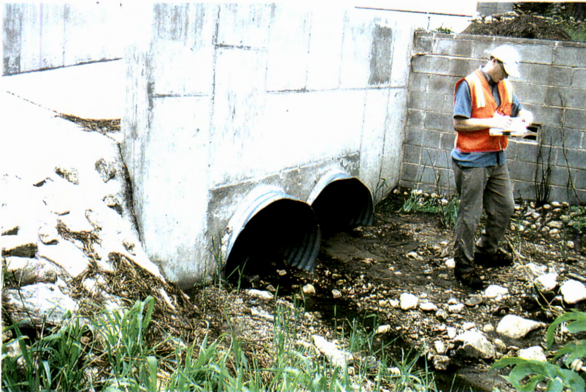
Picture 88. Downstream of culvert looking upstream at 2-36" CMPs (# 15).
