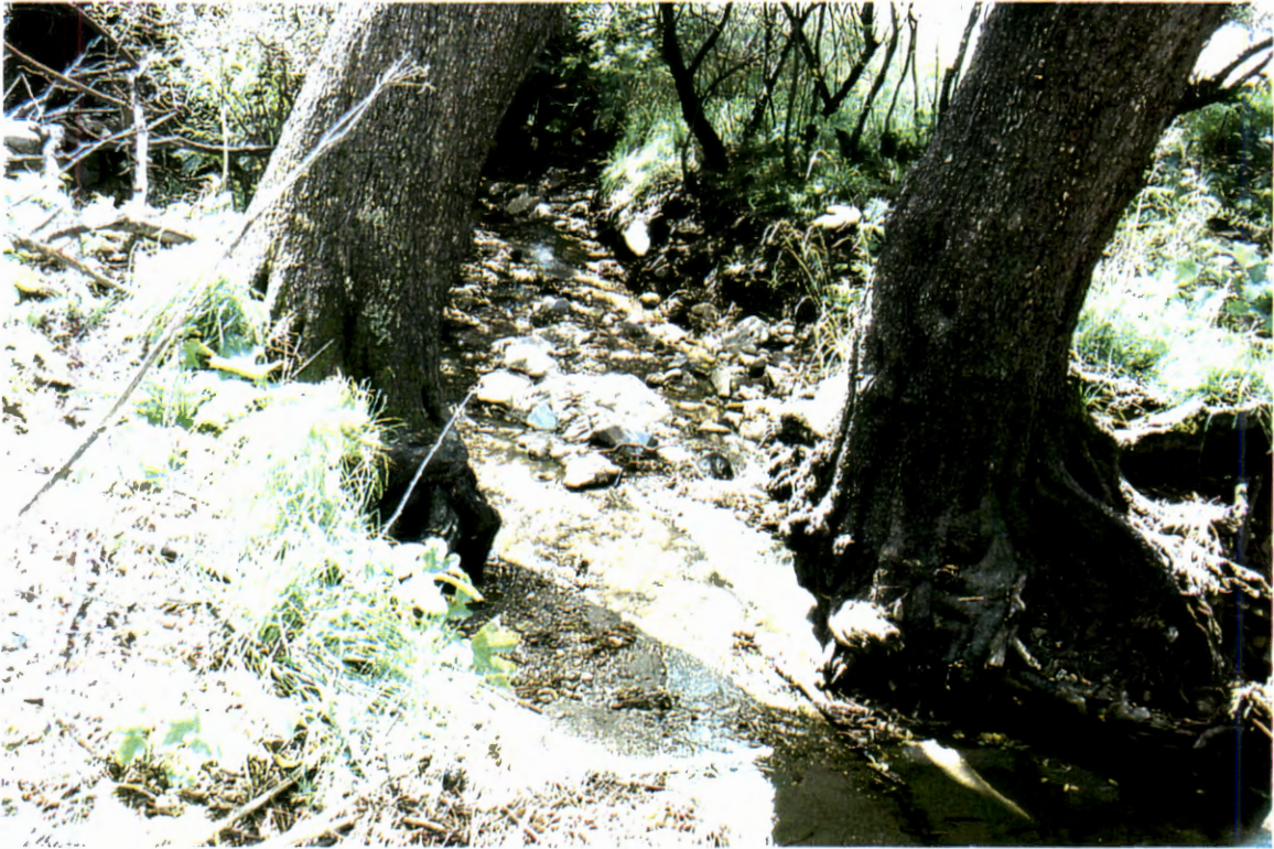
Picture 48. Top of driveway culvert (# 5) looking downstream at channel
