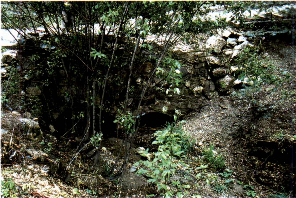
Picture 108. Upstream of driveway culvert looking downstream at 2- 4' x 6' ellipse CMPs (# 20).
