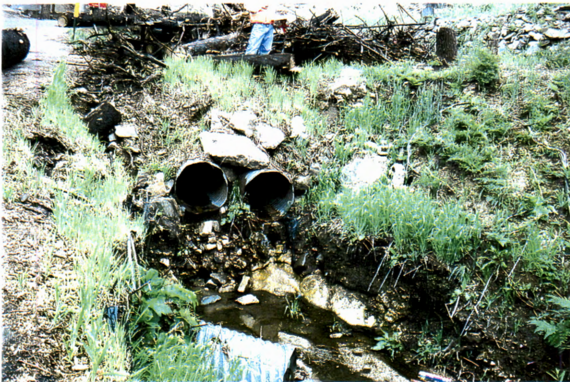
Picture 80. Downstream of culvert looking upstream at 2-36" CMPs (# 13).
