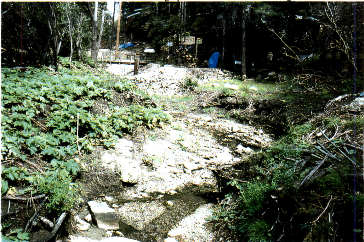
Picture 36. Upstream of dirt road crossing looking upstream at incised channel.
