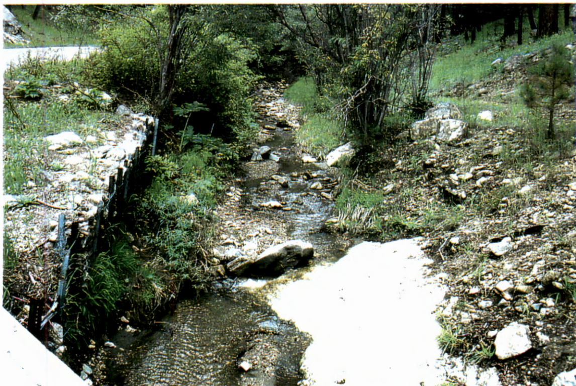
Picture 32. At East Sabino Road culverts (# 2) looking upstream at channel.
