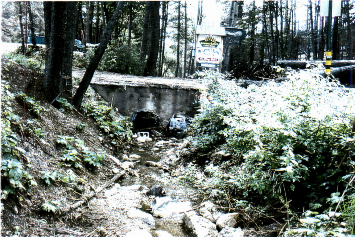
Picture 63. Upstream of coffee house driveway looking downstream at 2-40" CMPs (# 8).
