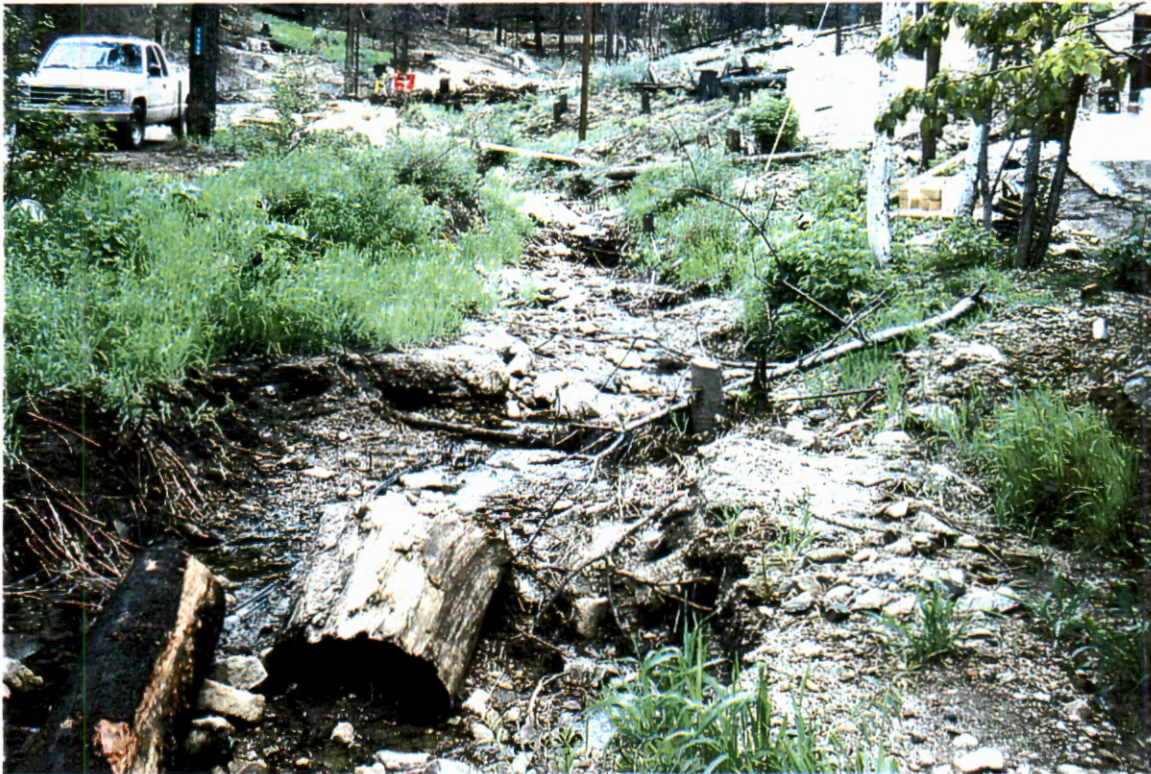
Picture 77. Centerline of driveway culvert (#12) looking upstream at centerline of channel.
