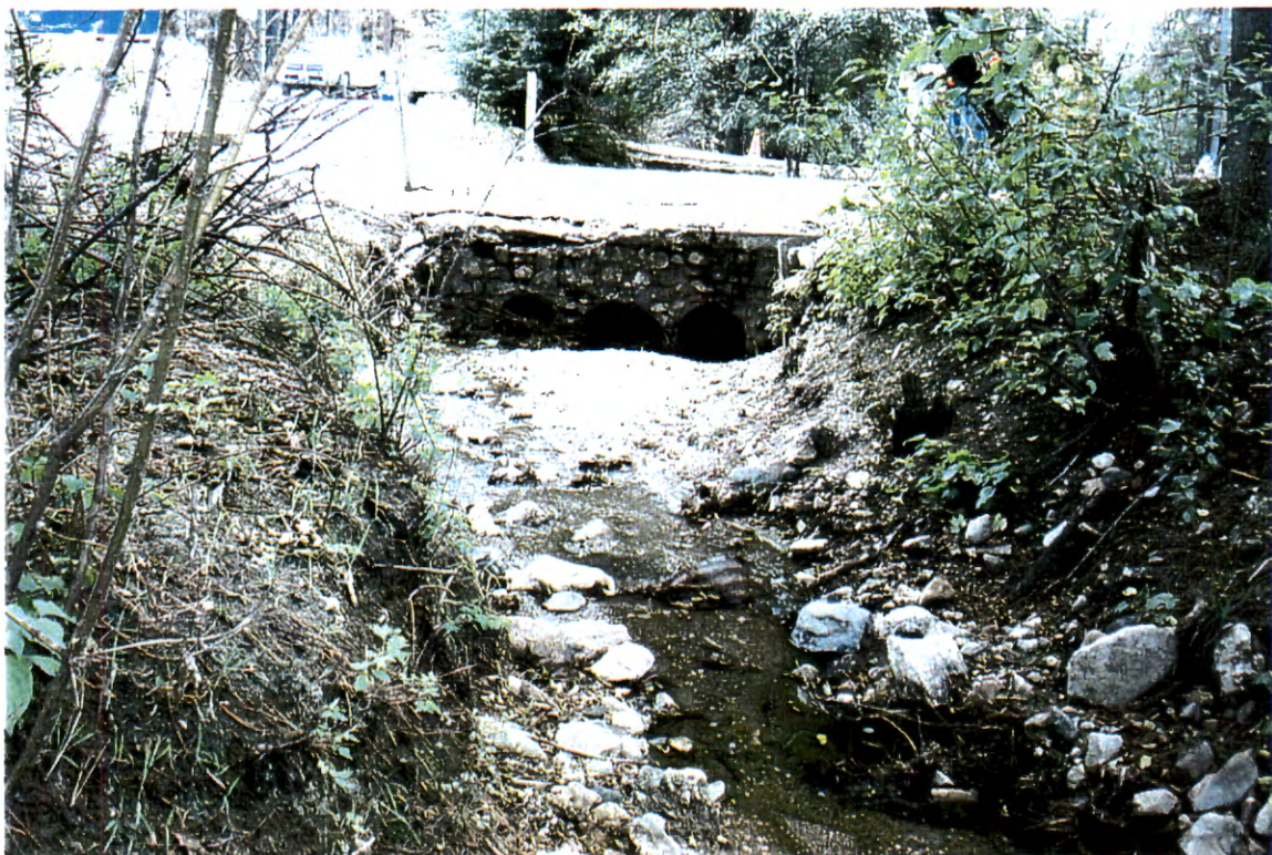
Picture 59. Upstream of driveway looking downstream at 2-24" and 1-36" CMPs (# 7).
