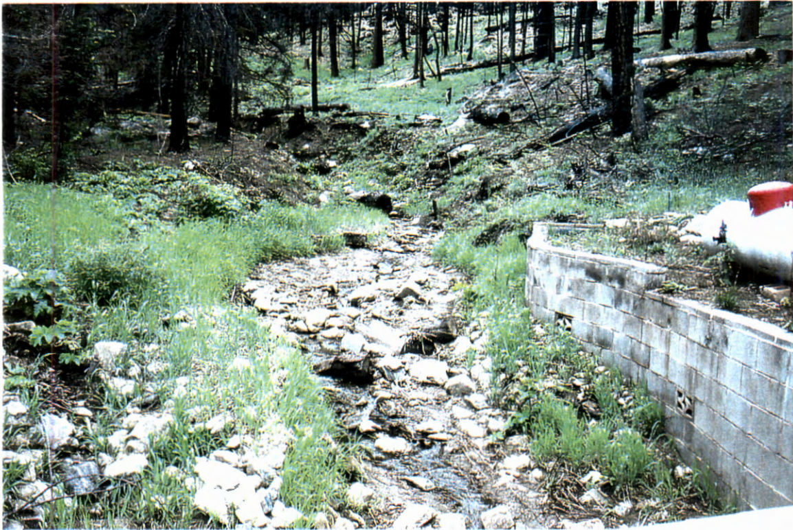
Picture 89. Centerline of driveway culvert (#15) looking upstream at centerline of channel.
