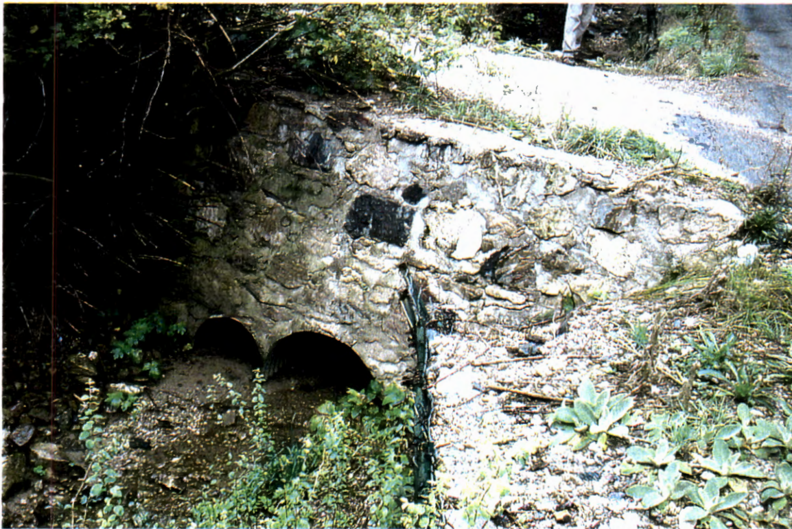
Picture 94. Downstream of driveway looking upstream at 36" CMP and 24" CMP (# 16).
