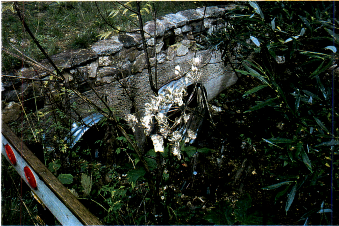
Picture 100. Upstream of driveway culvert looking downstream at 2-48" CMPs (# 18).
