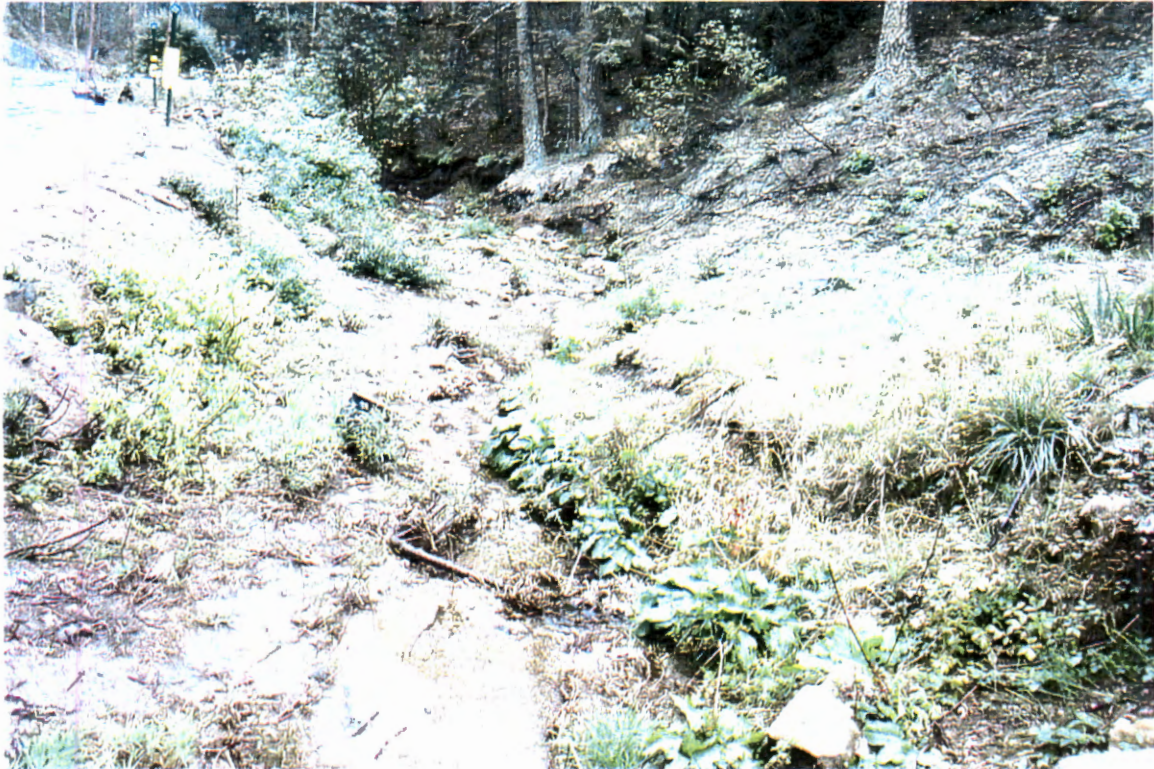
Picture 105. At driveway culvert (# 19) looking downstream at centerline of channel.
