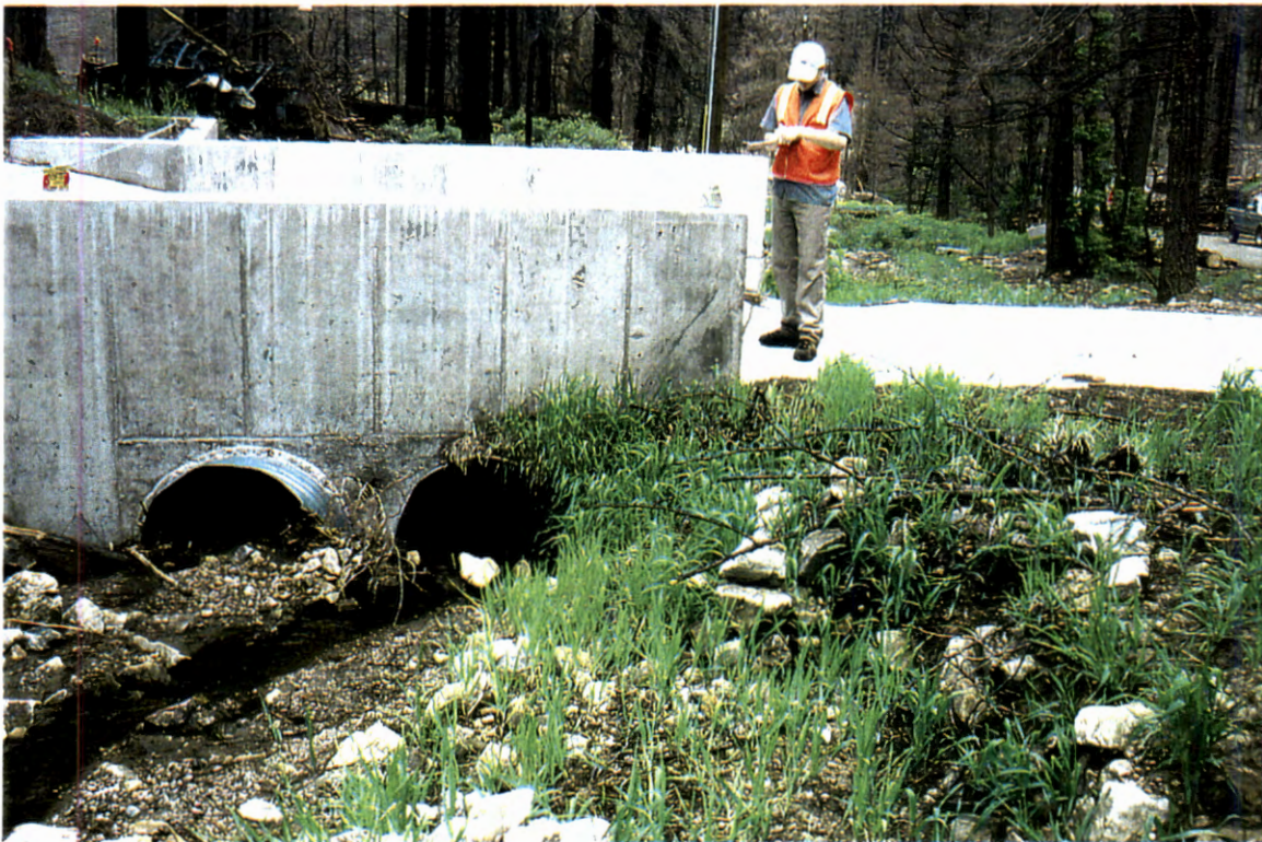
Picture 90. Upstream of driveway culvert looking downstream at 2-36" CMPs (# 15).
