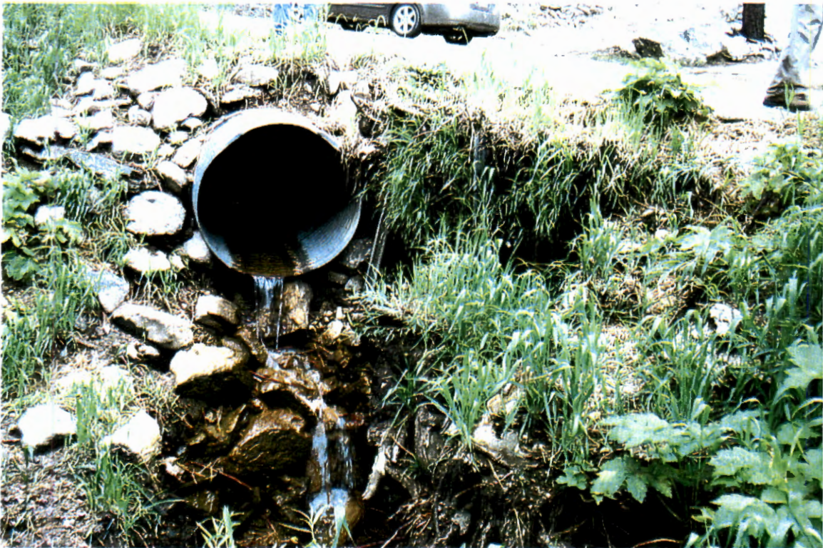
Picture 70. Downstream of Carter Canyon Road looking upstream at 42" CMP (# 10).
