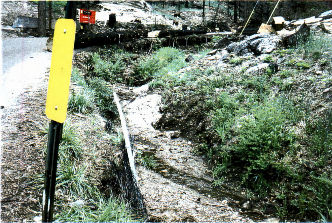
Picture 81. Upstream of culvert (#13) looking upstream at centerline of channel.
