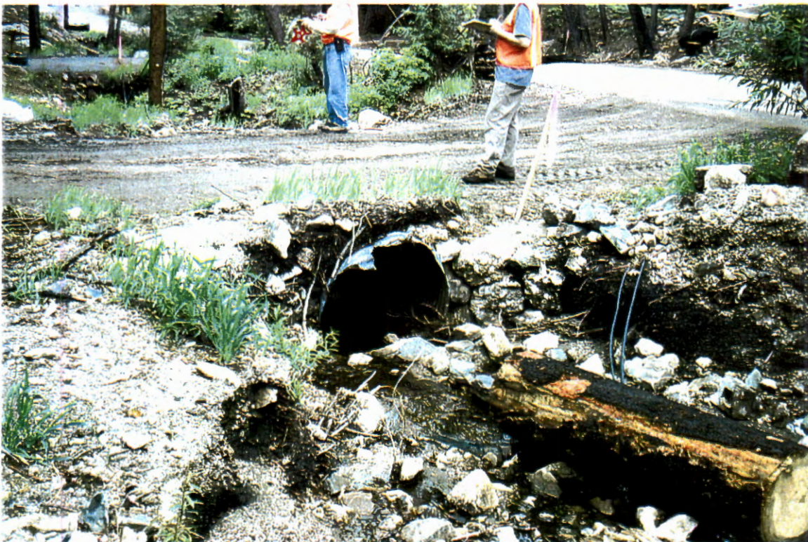
Picture 78. Upstream of driveway culvert looking downstream at 36" CMP (# 12).
