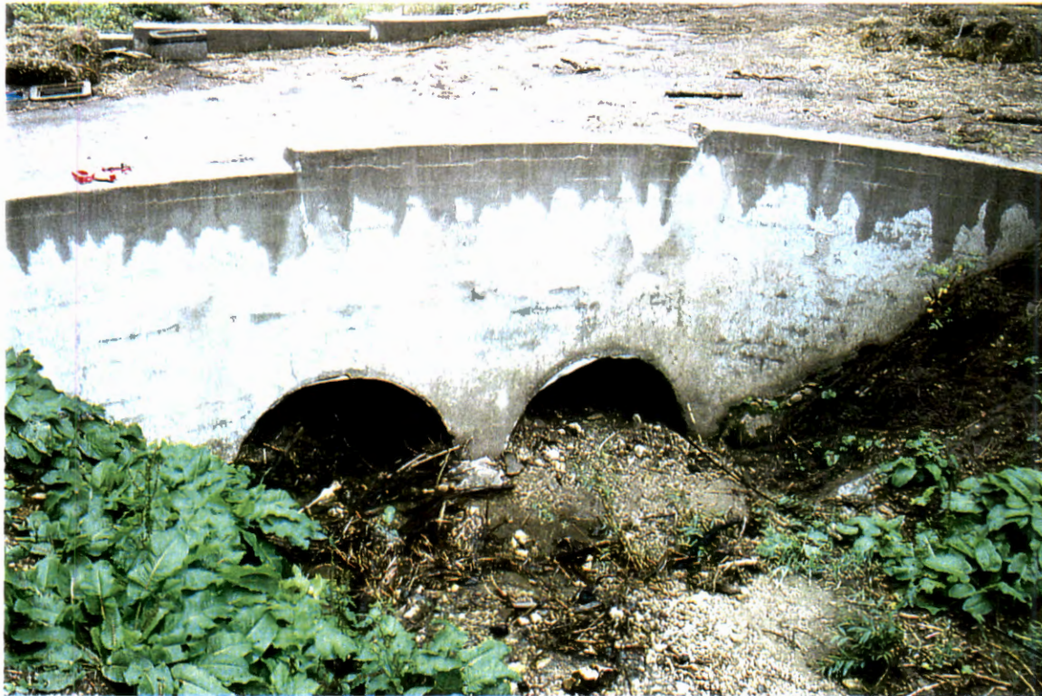
Picture 104. Upstream of driveway culvert looking downstream at 2-36" CMPs (# 19).
