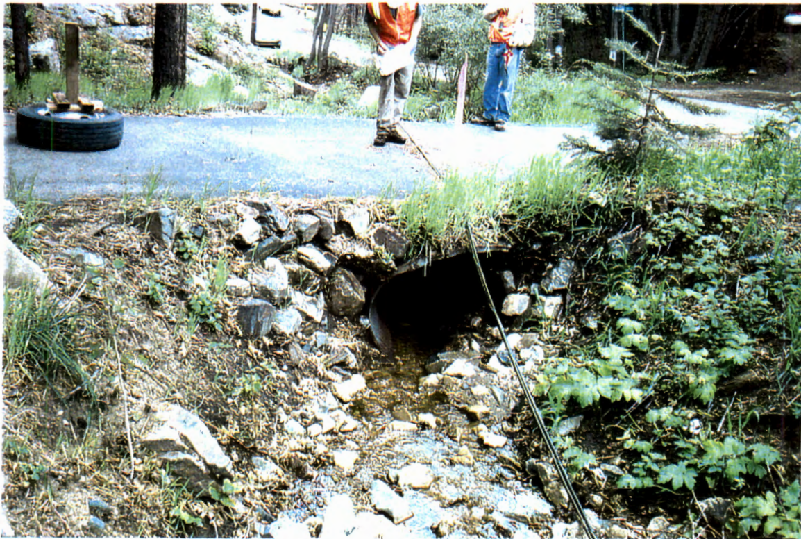
Picture 76. Upstream of driveway culvert looking downstream at 36" CMP (# 11).
