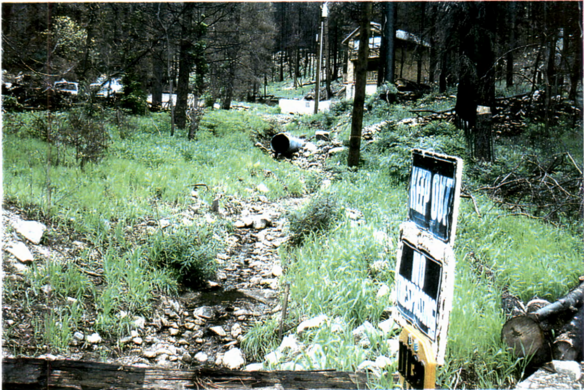
Picture 85. Centerline of driveway culvert (# 14) looking upstream at centerline of channel.
