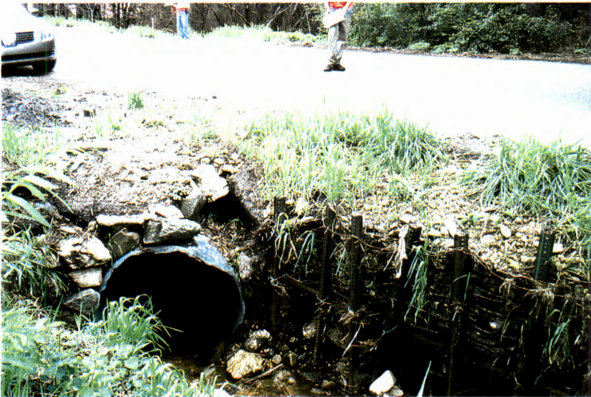
Picture 72. Upstream of Carter Canyon Road looking downstream at 42" CMP (# 10).
