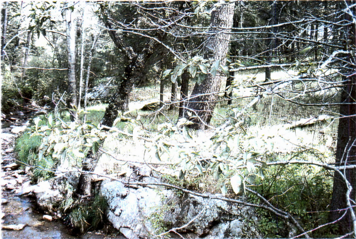
Picture 1. Downstream LOS looking upstream at rockwall protecting Marshall Gulch right parking lot.
