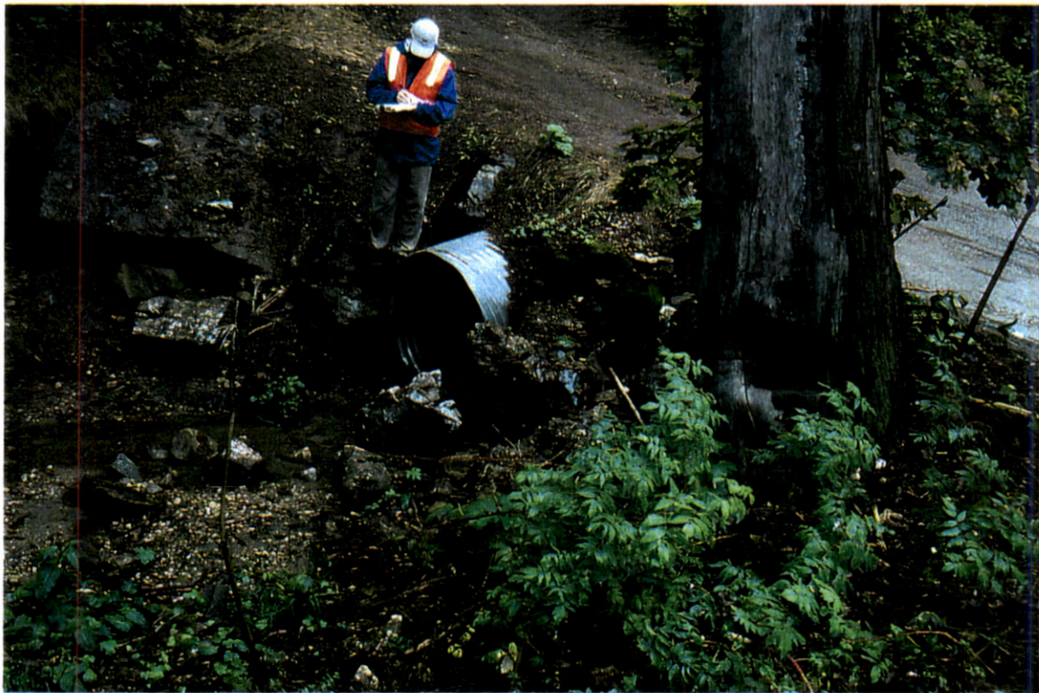
Picture 98. Downstream of Guthrie Road looking upstream at 36" CMP (# 17).
