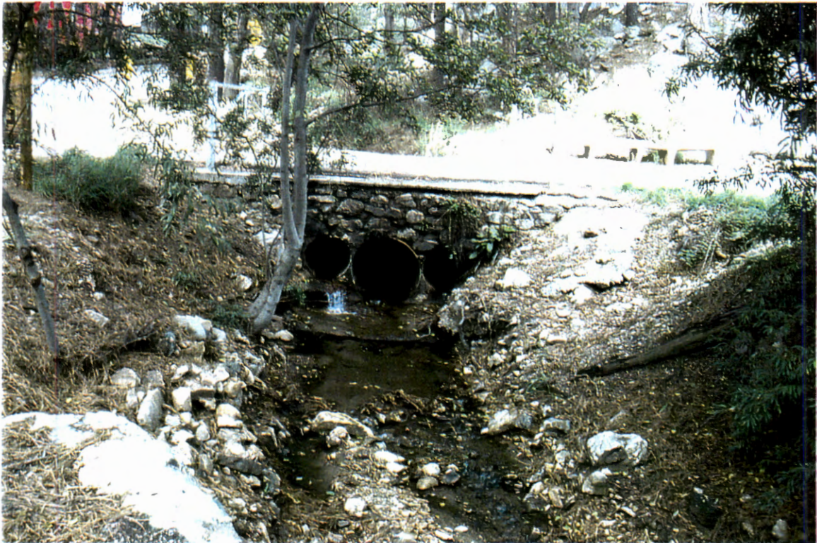
Picture 56. Top of driveway (# 6) looking upstream at 2-24" CMPs and 1-36" CMP (# 7).
