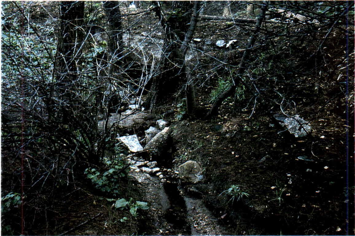
Picture 115. Downstream of 36" CMP on Tucson Road looking upstream at CMP (# 21).
