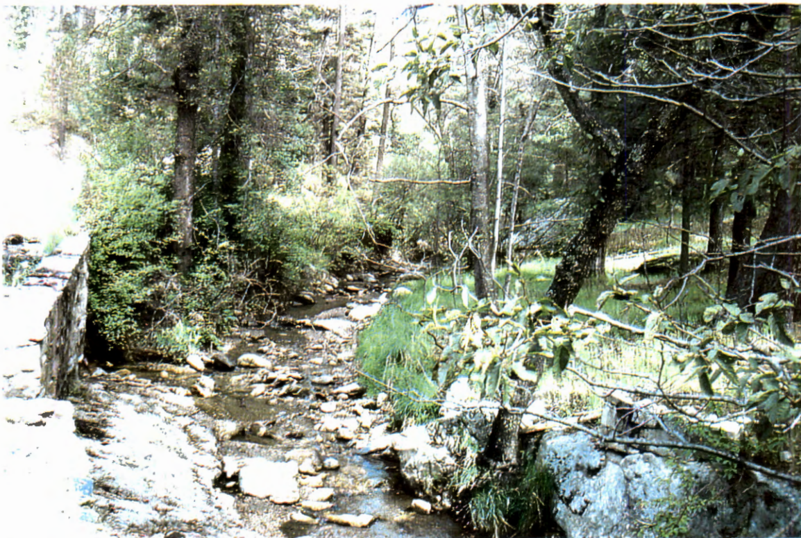
Picture 2. Downstream LOS looking upstream at rockwall and channel.
