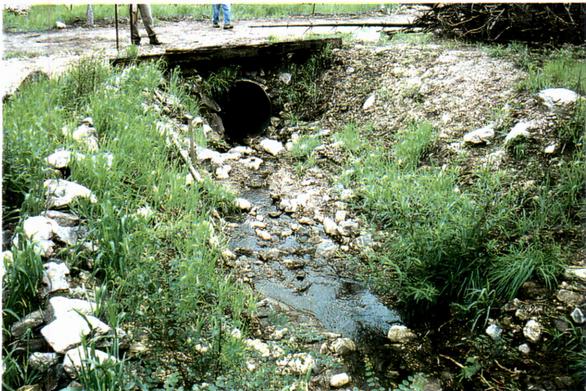
Picture 86. Upstream of driveway culvert looking downstream at 36" CMP (# 14).
