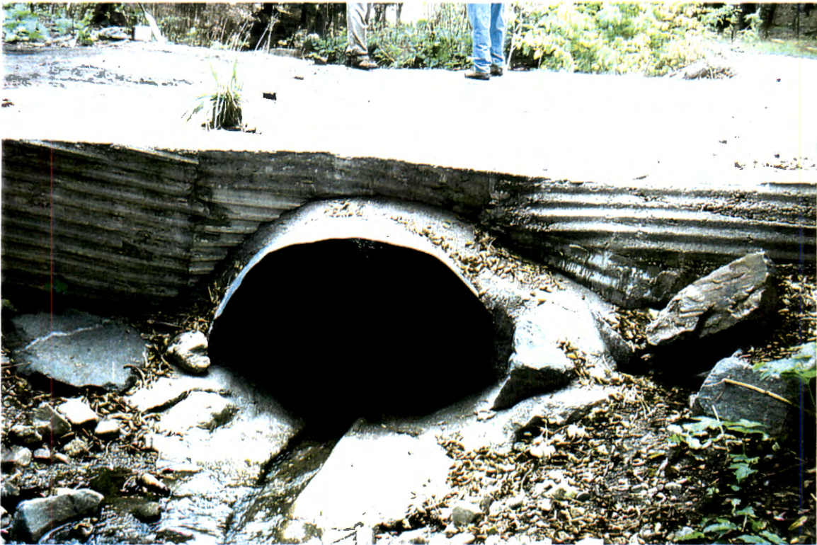
Picture 44. Upstream of driveway culvert looking downstream at elliptical culvert (# 3).
