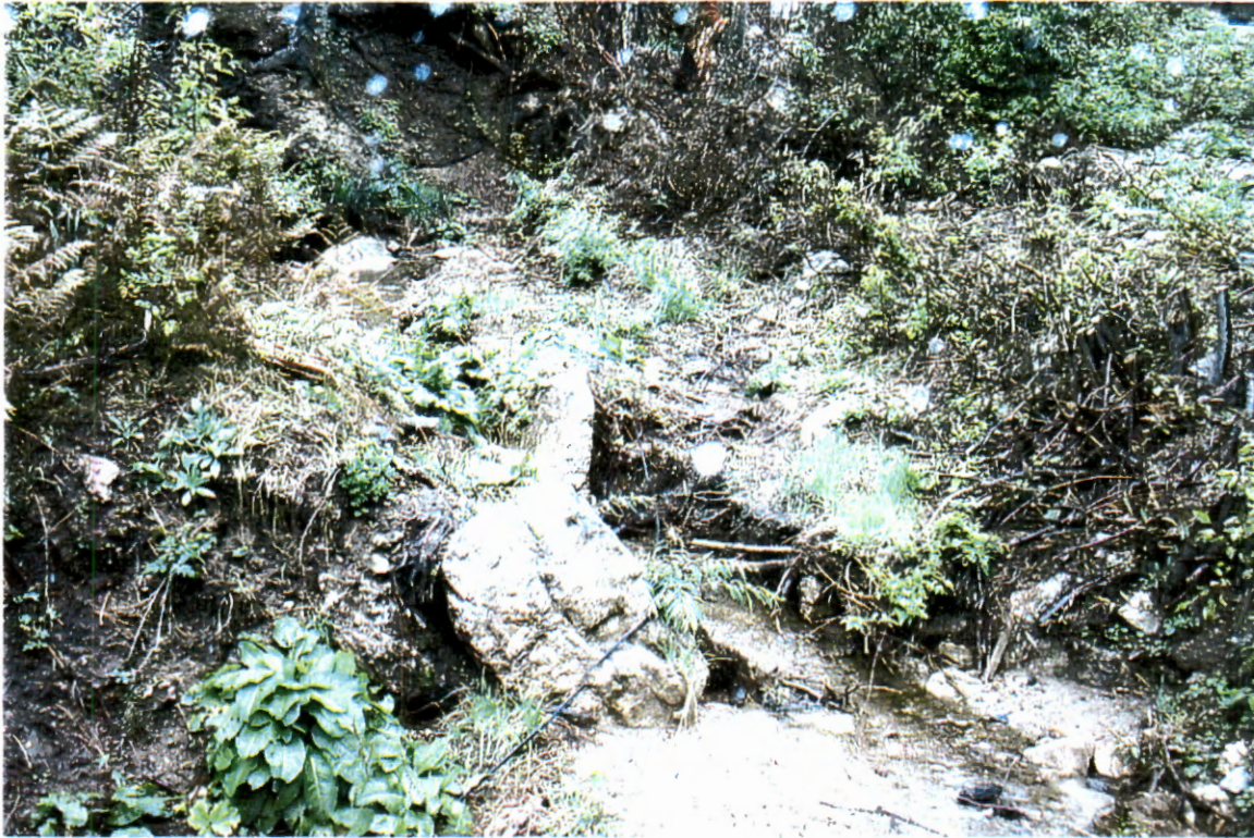
Picture 103. At driveway culvert (# 19) looking upstream at centerline of channel.
