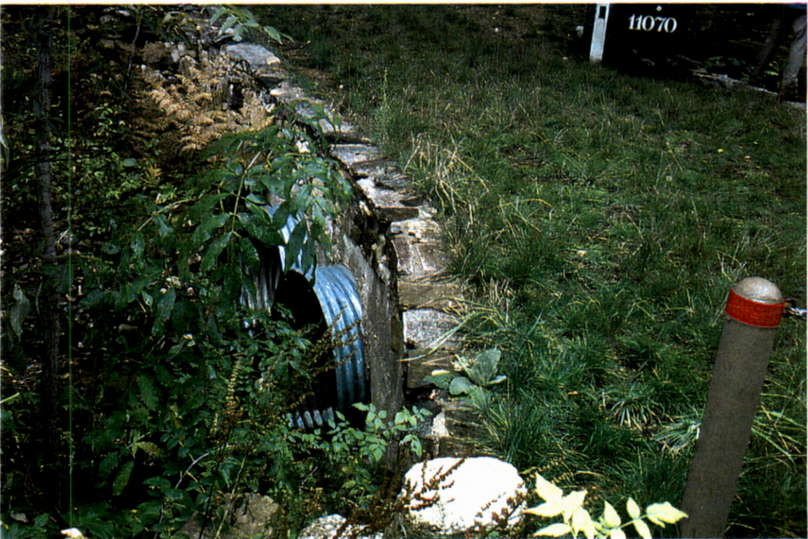
Picture 102. Downstream of driveway culvert looking upstream at 2-48" CMPs (# 18).
