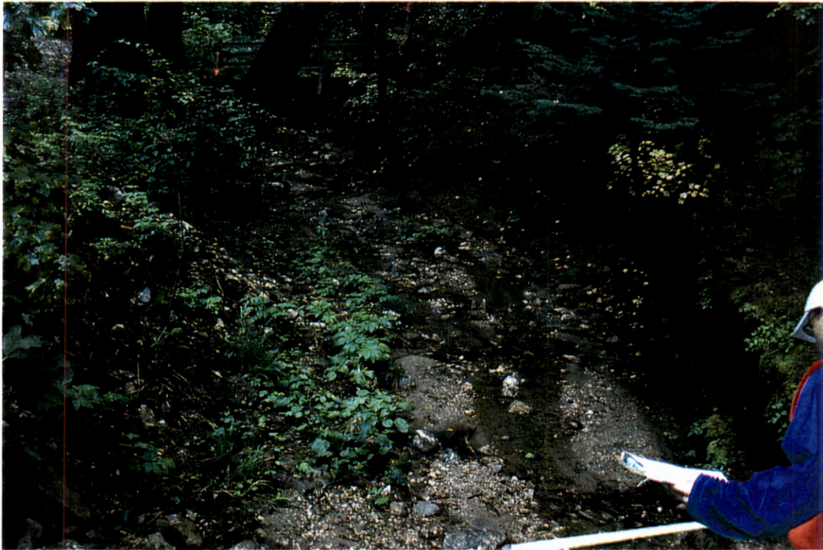
Picture 97. At Guthrie Road culvert (#17) looking downstream at channel.
