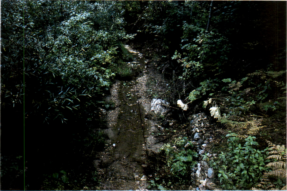
Picture 101. At driveway culvert (# 18) looking downstream at centerline of channel.
