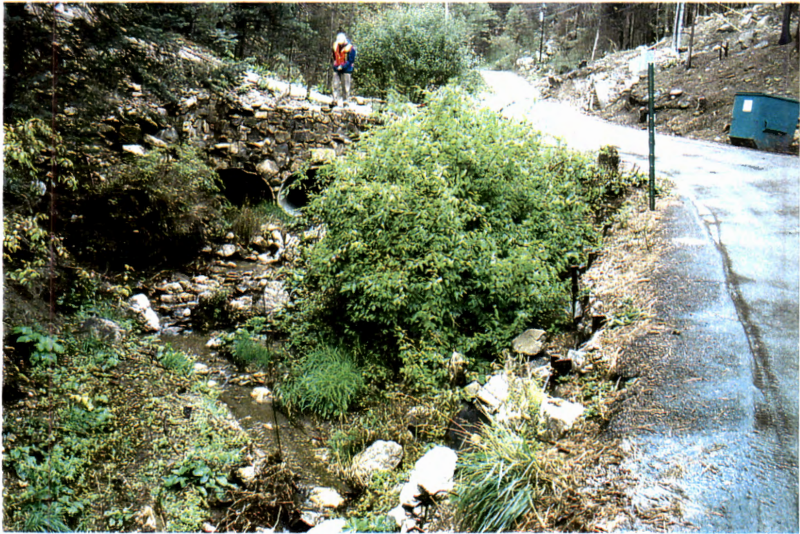
Picture 110. Downstream of driveway culvert looking upstream at two ellipse CMPs (# 20).
