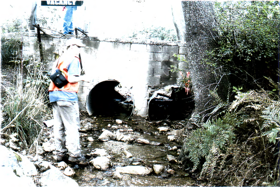
Picture 61. Downstream of coffee house driveway looking upstream at 2-40" CMPs (# 8).
