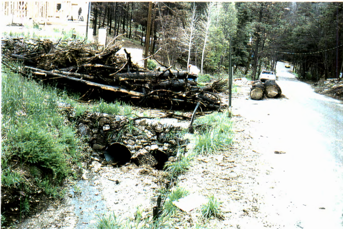
Picture 82. Upstream of culvert looking downstream at 2-36" CMPs (# 13).
