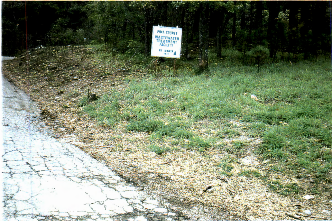
Picture 38. Pima County Waste Water Treatment Facility.
