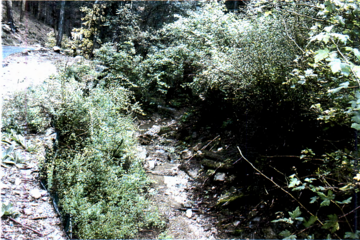
Picture 93. From driveway culvert (#16) looking downstream at channel.
