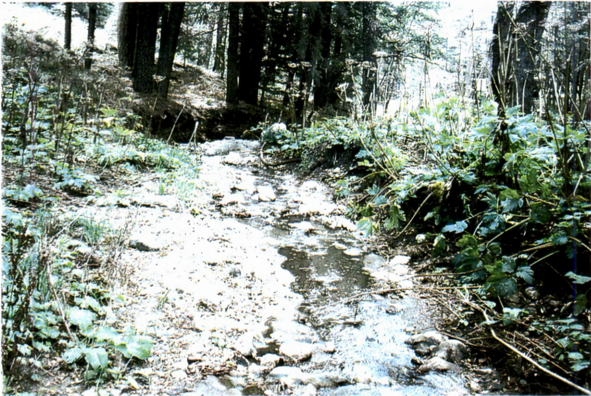
Picture 41. Downstream of driveway culvert (# 3) looking downstream at channel.
