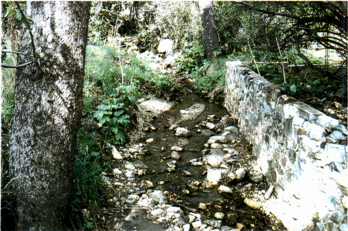
Picture 50. Top of driveway culvert (# 5) looking upstream at channel.
