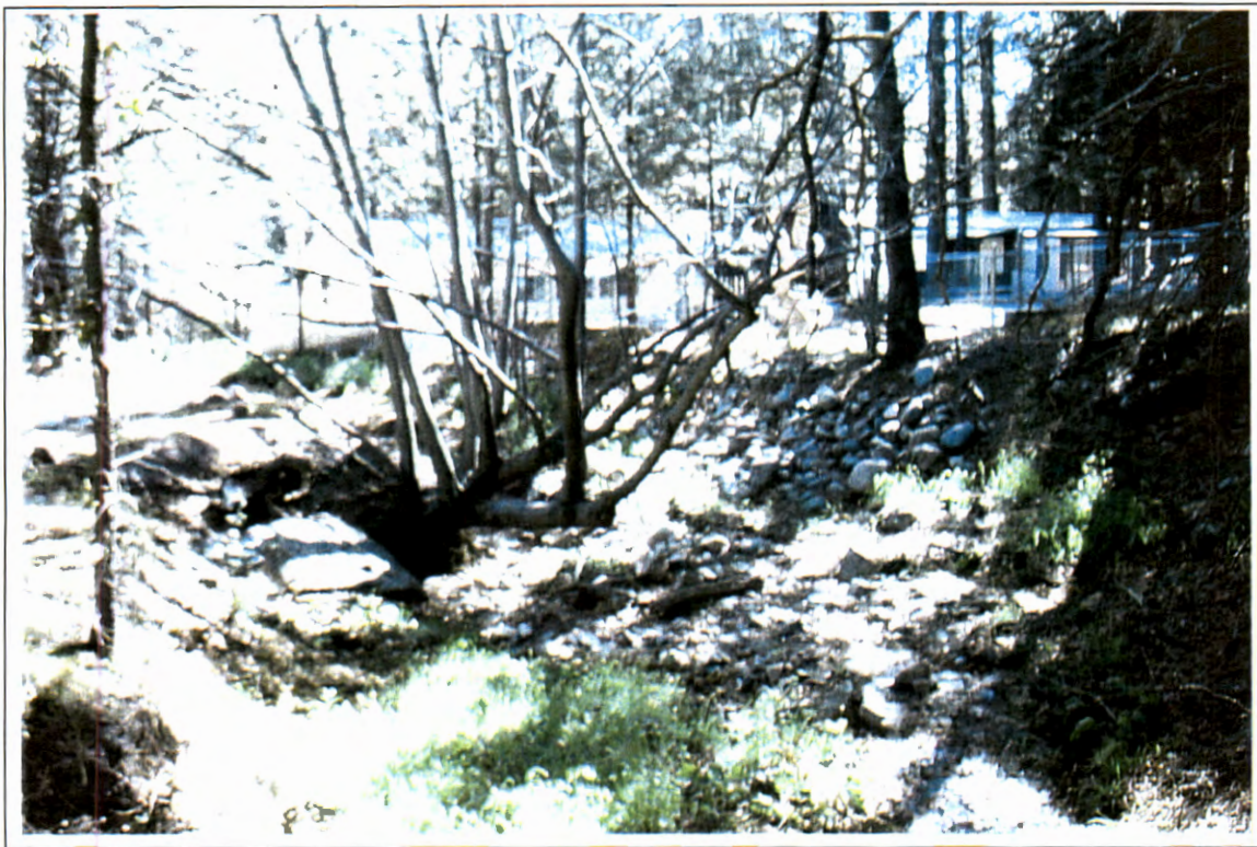
PHOTOGRAPH 124 – Looking downstream at Carter Canyon. Zimmerman Elementary school is in the background. Notice rock placement at streambank to protect school grounds.
