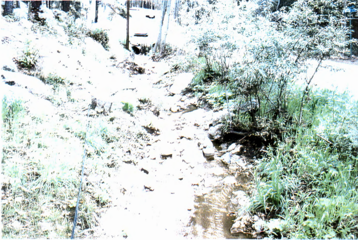
Picture 73. Centerline of driveway culvert looking downstream at centerline of channel.
