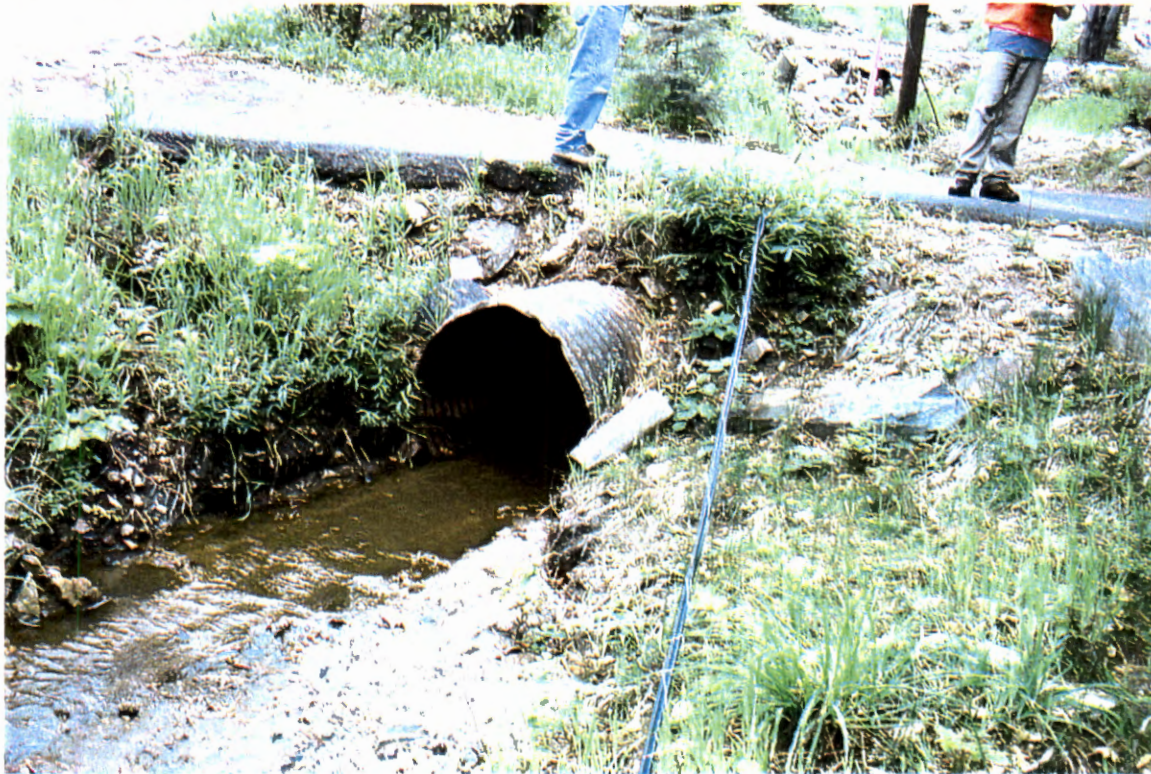
Picture 74. Downstream of driveway culvert looking upstream at 36" CMP (# 11).
