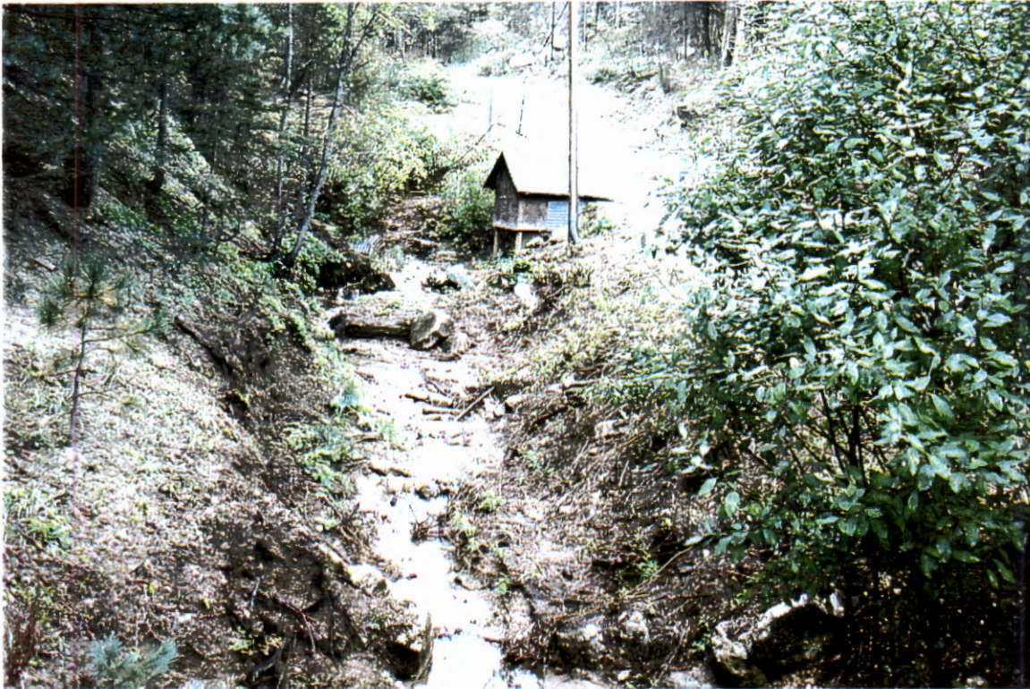
Picture 107. At driveway culvert (#20) looking upstream at centerline of channel.
