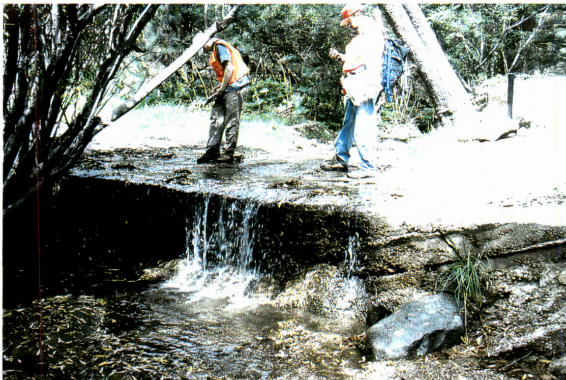
Picture 39. Downstream of driveway crossing looking upstream at 2.5' drop on the downstream side of driveway.
