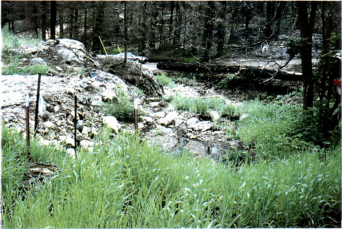
Picture 83. Centerline of driveway culvert (# 14) looking downstream at centerline of channel.
