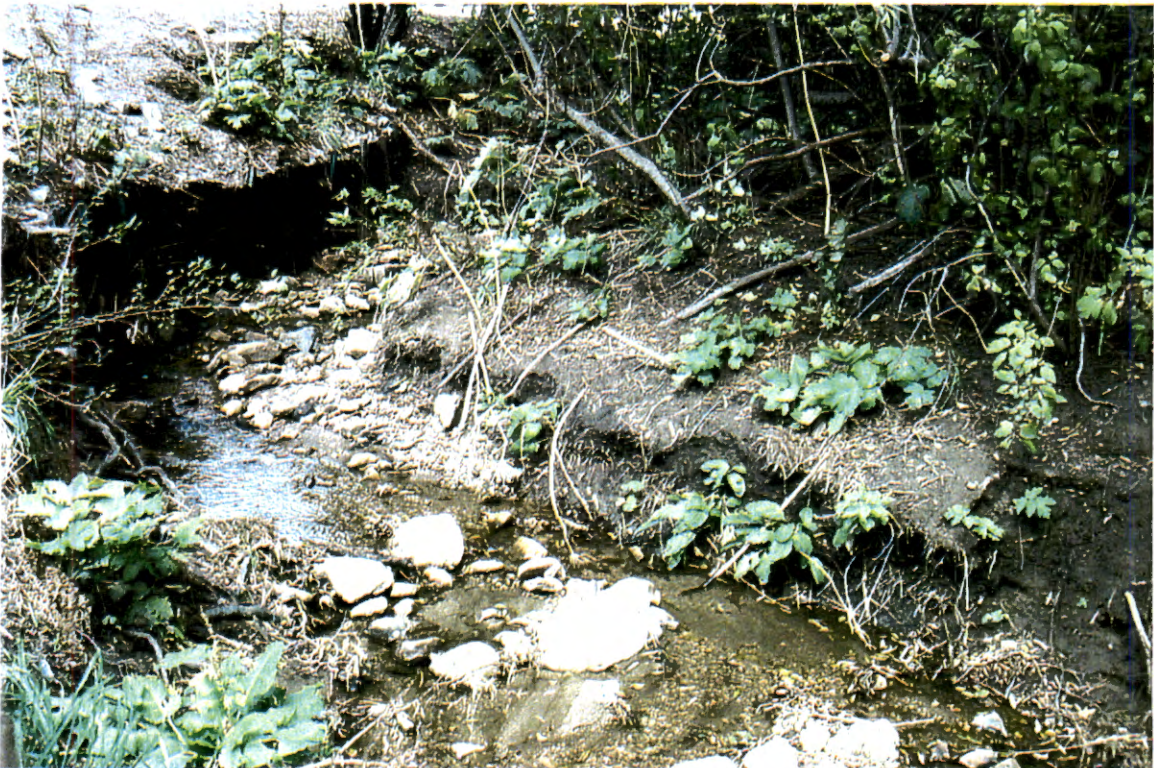
Picture 46. Upstream of Goat Hill Road culvert (# 4) looking upstream at channel.
