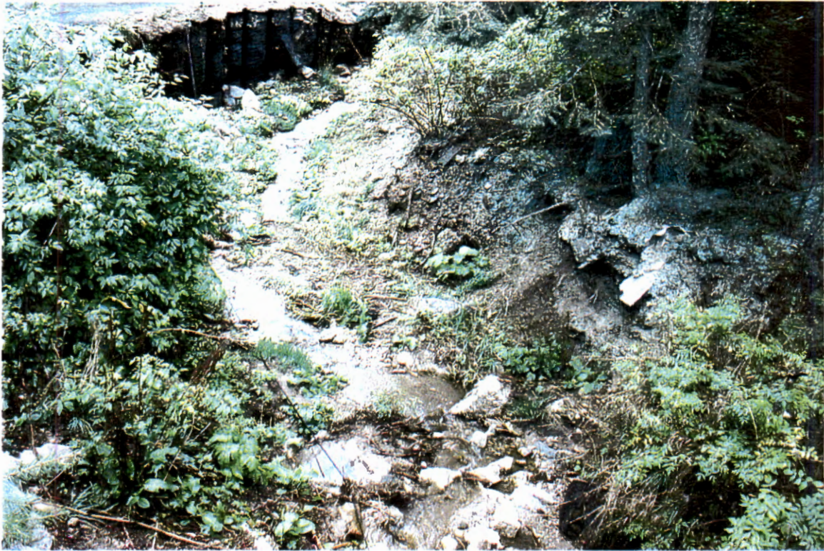
Picture 109. At driveway culvert (# 20) looking downstream at centerline of channel.
