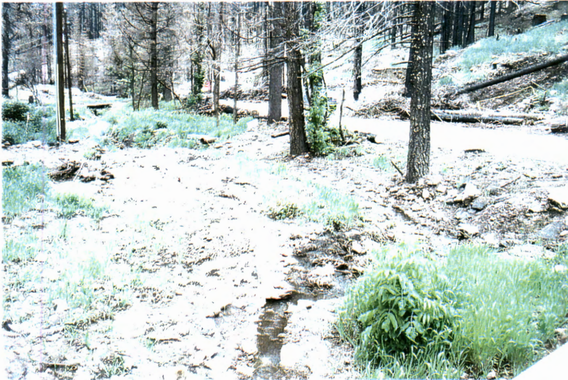
Picture 87. Centerline of driveway culvert (#15) looking downstream at centerline of channel.
