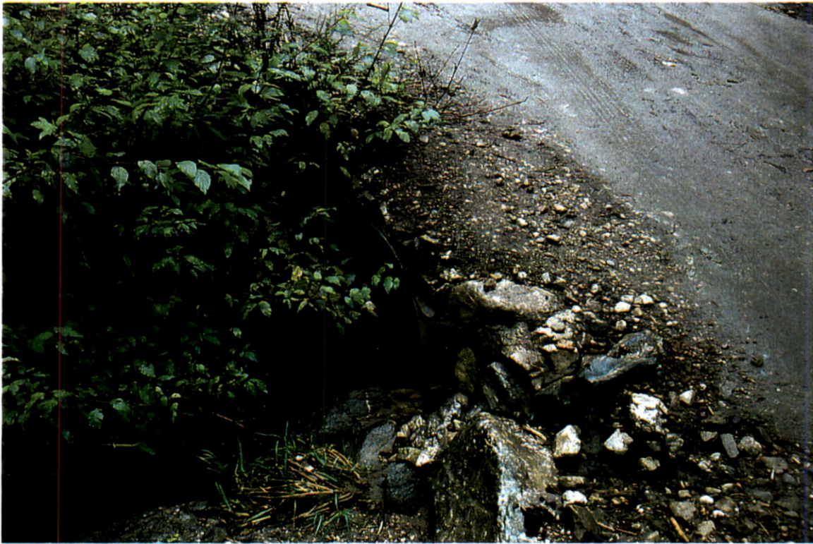
Picture 96. Upstream of Guthrie Road looking downstream at 36" CMP (# 17).
