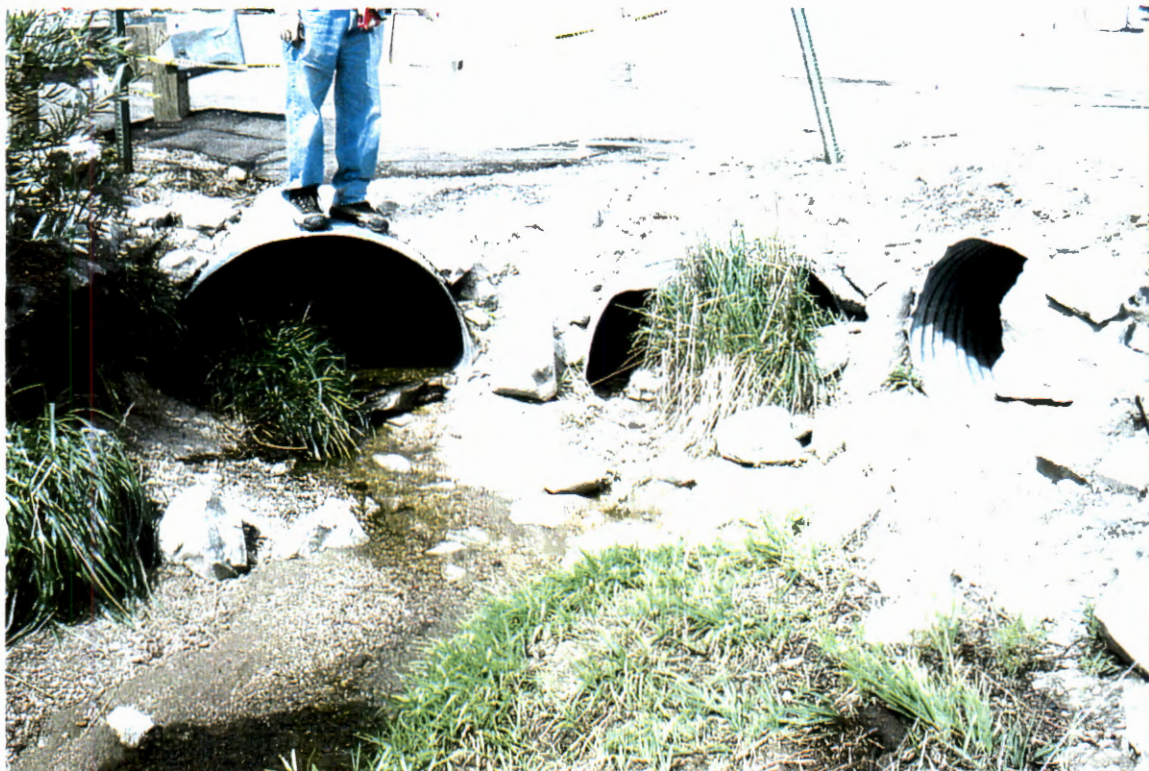
Picture 65. Downstream of Sabino Canyon Road looking upstream at elliptical culvert (# 9).
