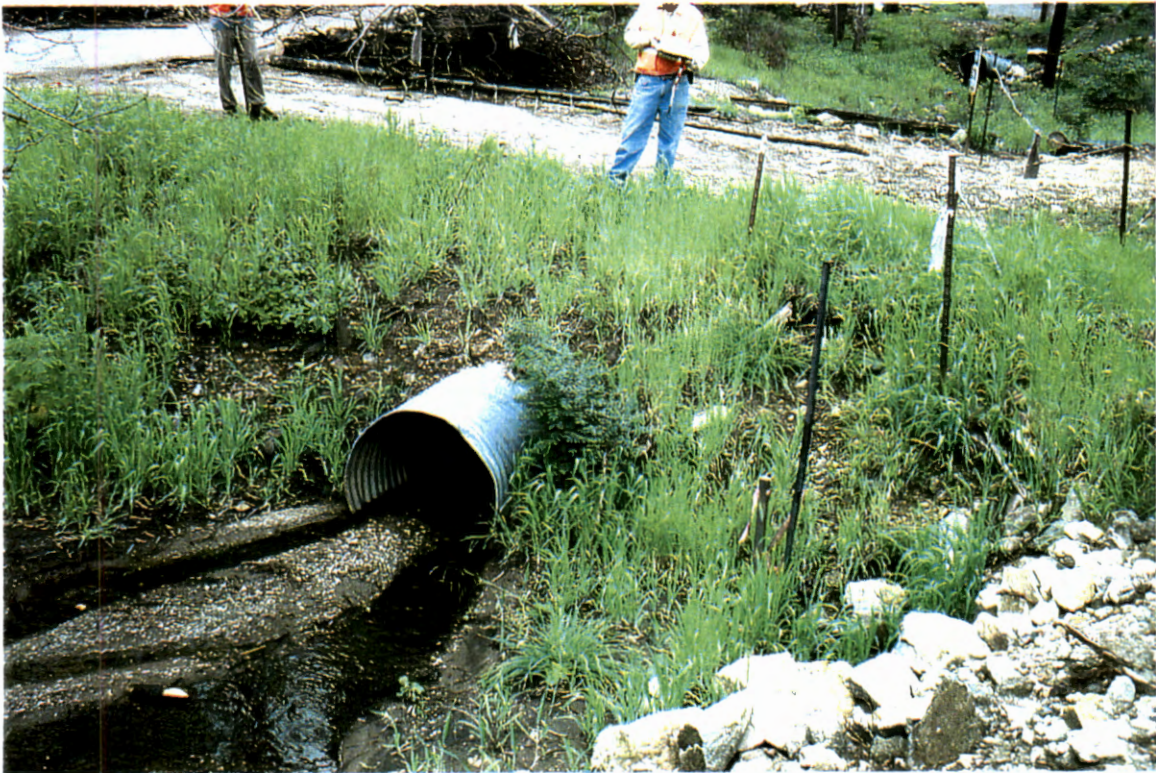
Picture 84. Downstream of driveway culvert looking upstream at 36" CMP (# 14).
