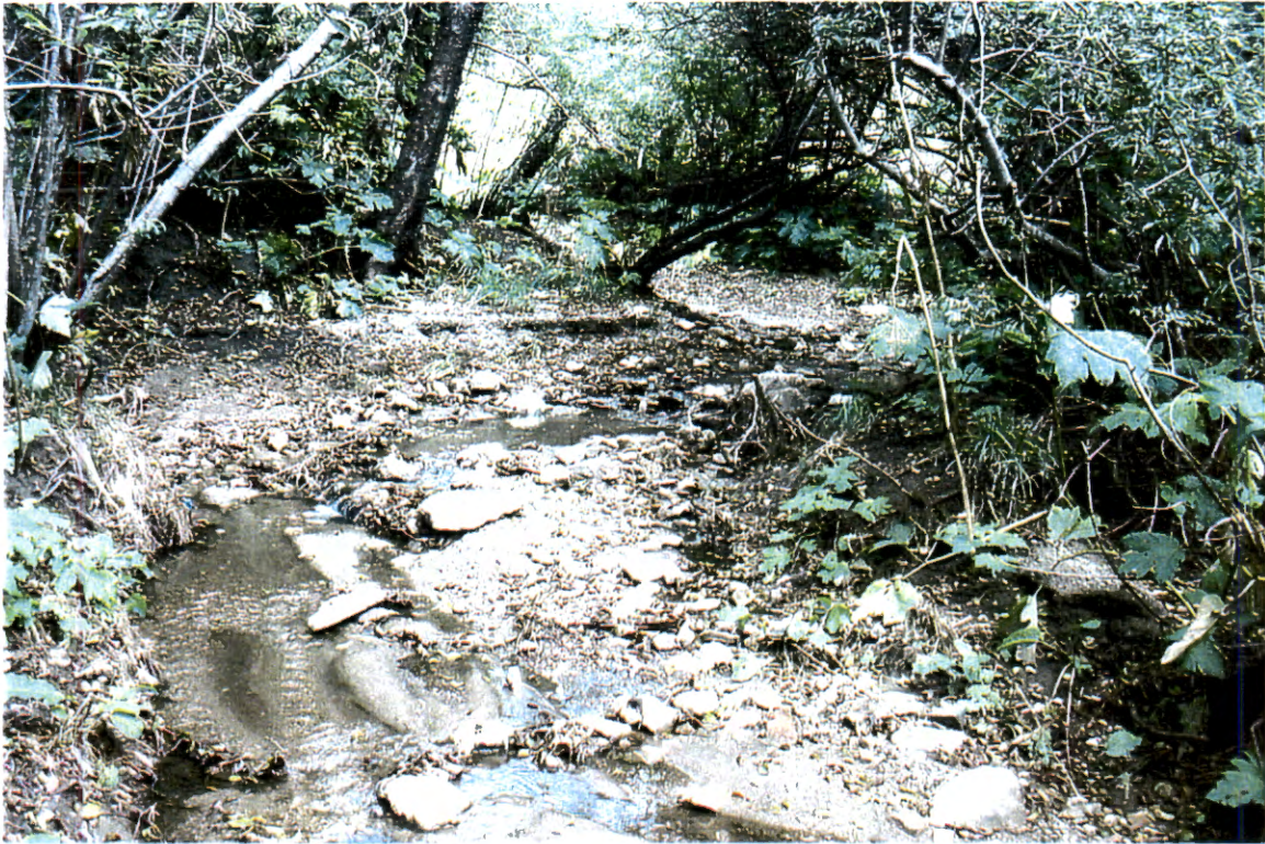
Picture 43. Upstream of driveway culvert (# 3) looking upstream at channel
