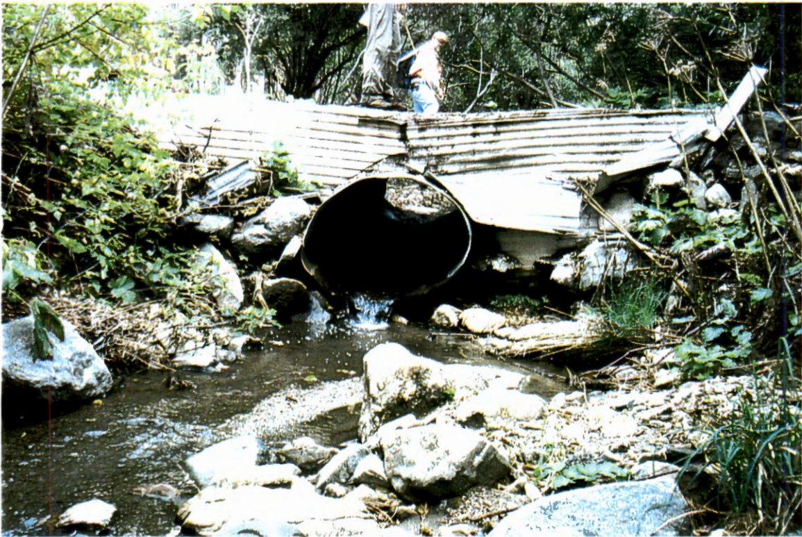
Picture 42. Downstream of driveway culvert looking upstream at elliptical CMP culvert (# 3).
