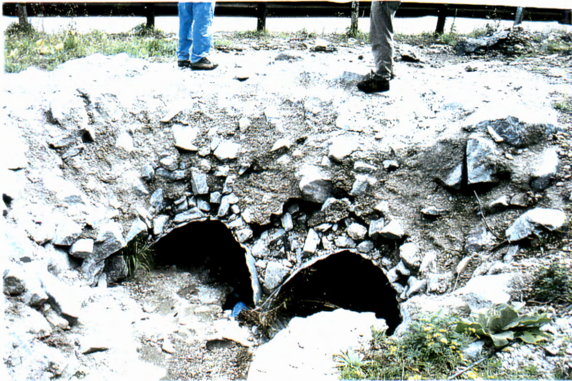
Picture 67. Upstream of Sabino Canyon Road looking downstream at elliptical culvert (# 9).
