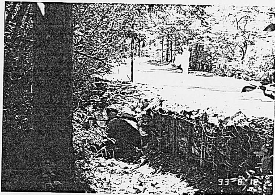
Upstream of crossing from the north to the south side of Carter Canyon Road (located at 11229 Carter Canyon Road).
