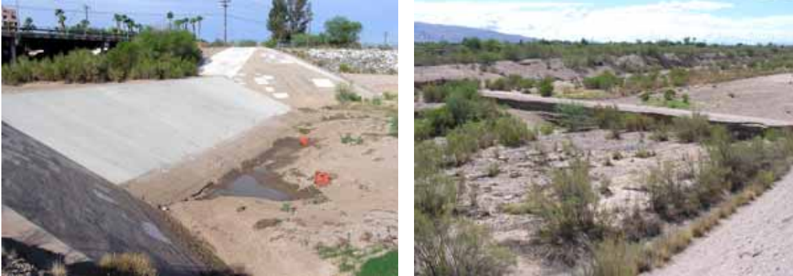
Figure 15. Grade control structures with scour pools supporting breeding amphibians in Pantano Wash, at Broadway (5 species, left) and about 0.6 mi upstream (1 species, right).
