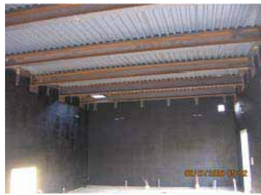
Roof Decking at TPSS No. 6
