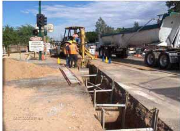
KWC Excavating for the new 12-inch private irrigation crossing 11 th Avenue
