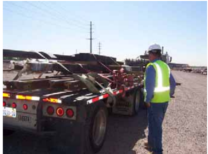
MP9 - 100 Meter Left Hand Crossover (4-9/4-10) being delivered to the MSF Storage Yard
