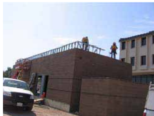
Parapet Framing at TPSS No. 1
