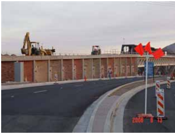
Southeast Retaining Wall
