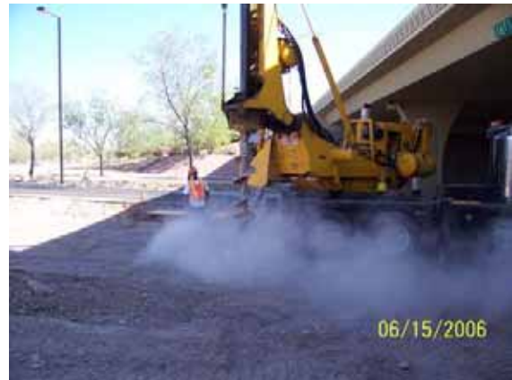
OCS foundation construction at SR202
