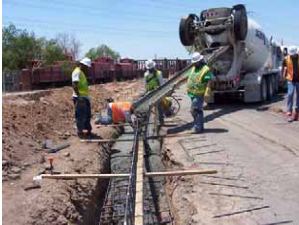
Retaining Wall 5, Ash to First Street
