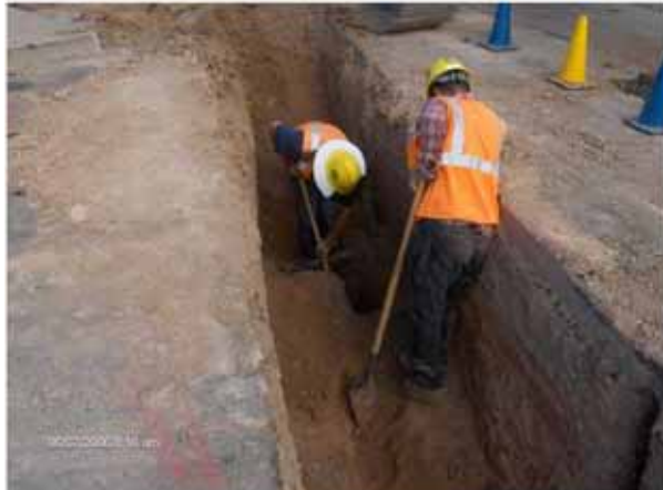
KWC laborer backfilling the CB-N16A Station 325+72.7 70.65 RT
