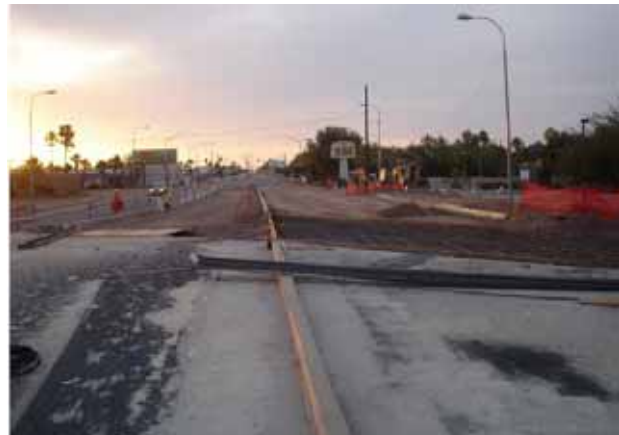
Roadway Work—East from Tempe Canal Bridge
