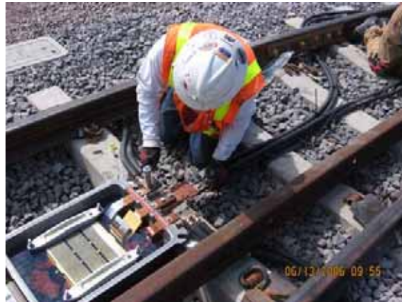
MSF Yard Installation of Impedance Bonds
