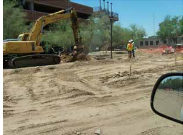
Roadway Work, Veterans' Way
