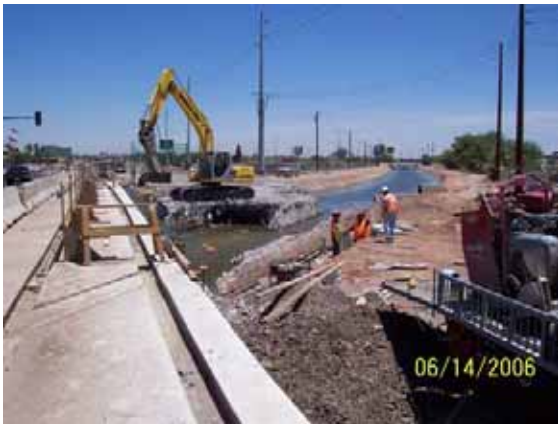
Demolition of the Washington Street bridge over the Grand Canal
