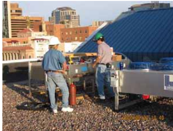
OCC Installation of HVAC Condenser Units
