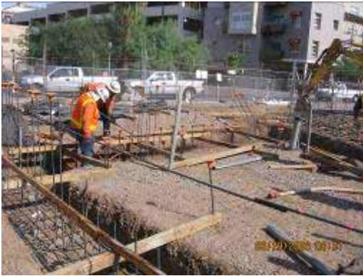
Installation of Rebar for TPSS No. 5 Footings
