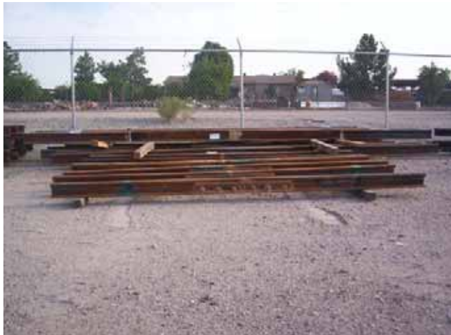
Bonded insulated joint delivery
