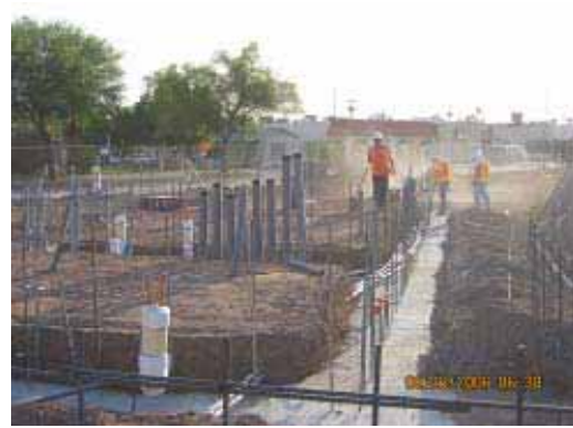
Footings at TPSS No. 7
