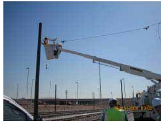
Installation of Headspan - North MSF Yard
