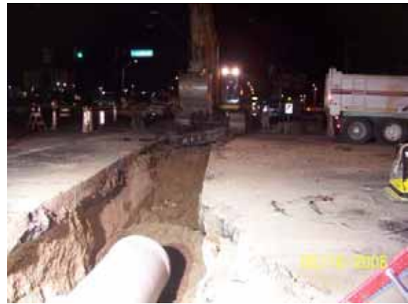
SRP irrigation installation at 40 th and Washington Streets
