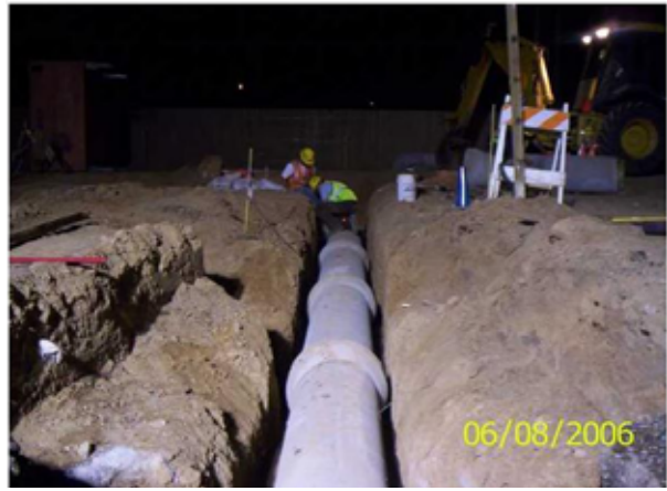
KWC crews installing a storm drain lateral at Sta. 463+80
