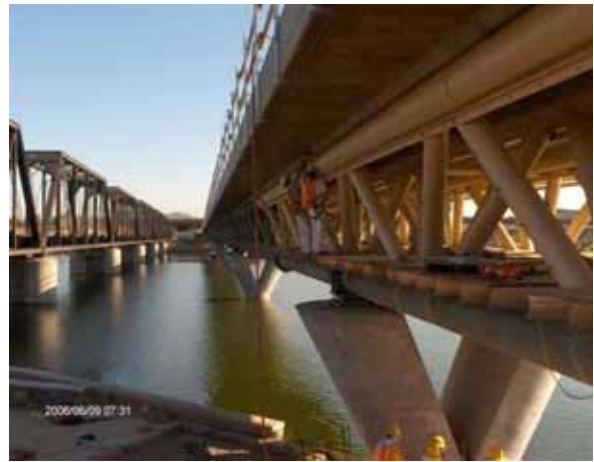
Painters Coating Trusses
