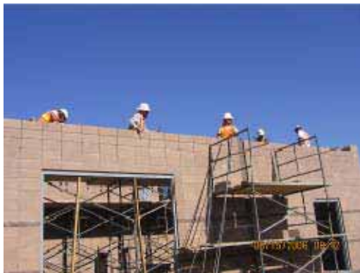
CMU Installation at TPSS No. 2
