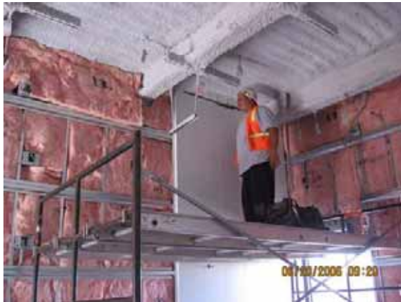
SB No. 5 Metal Liner Panels Installation
