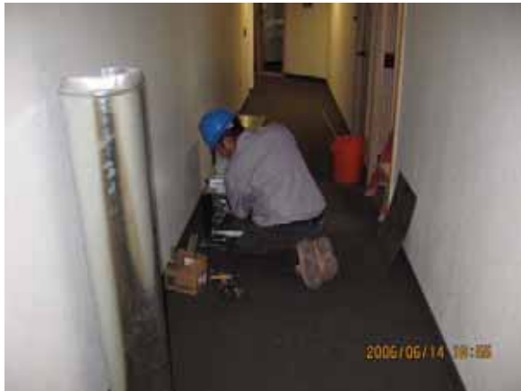
OCC - Installation of Mechanical Rough-In
