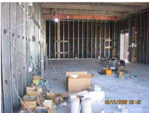
Electrical Rough-In at TPSS No. 15
