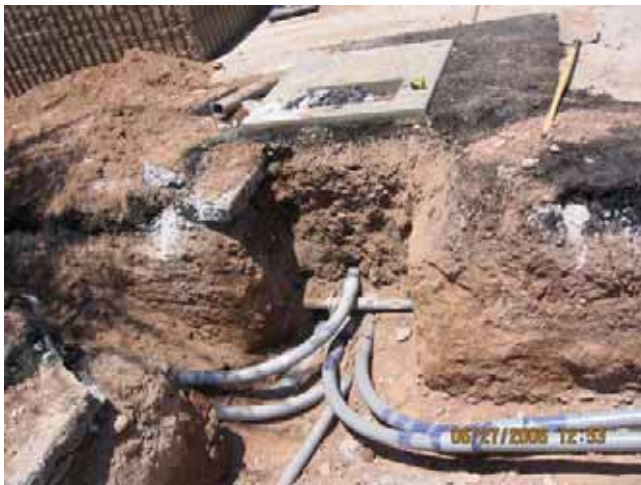
Installing APS conduit and transformer pad
