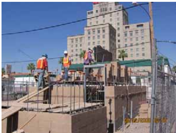
SB No. 3 Installation of 2 nd Masonry Lift
