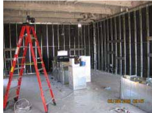
Electrical Rough-In at TPSS No. 8
