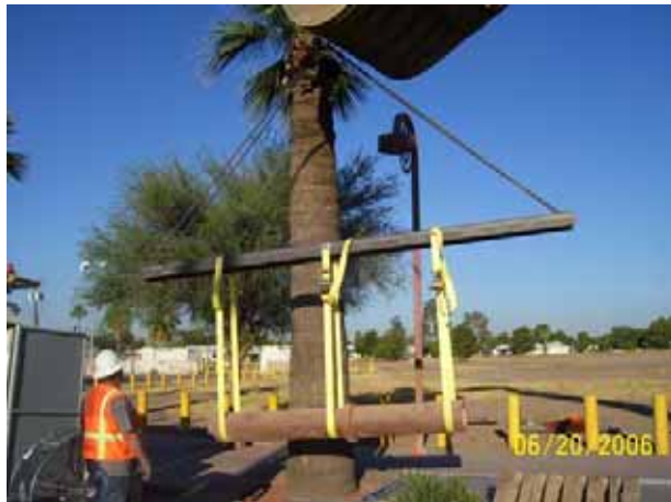
Installing Pipe near Steele/Indian School Park
