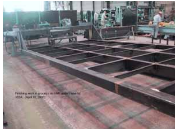
Finishing Work in process on METRO Underframe.
