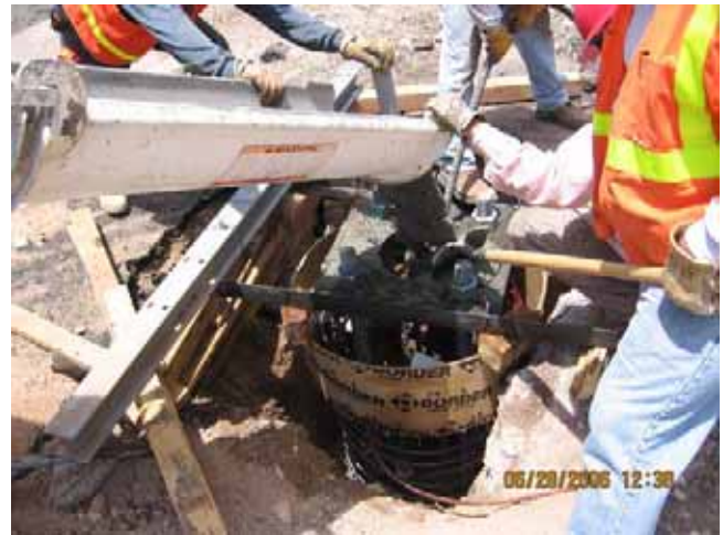
Placing Concrete at OCS Foundation
