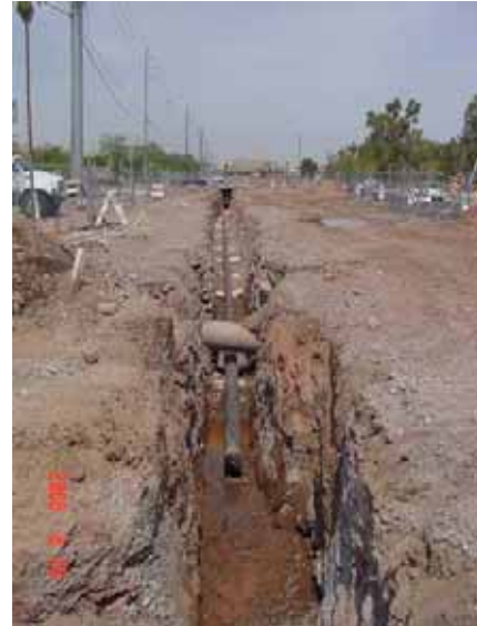
SWG relocating gas main on Washington Street Line Section 4
