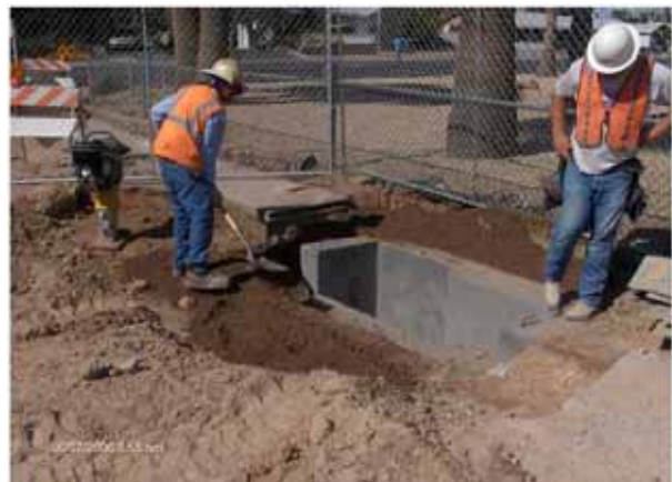
KWC laborer backfilling the CB-N16A Station 325+72 70.65 RT
