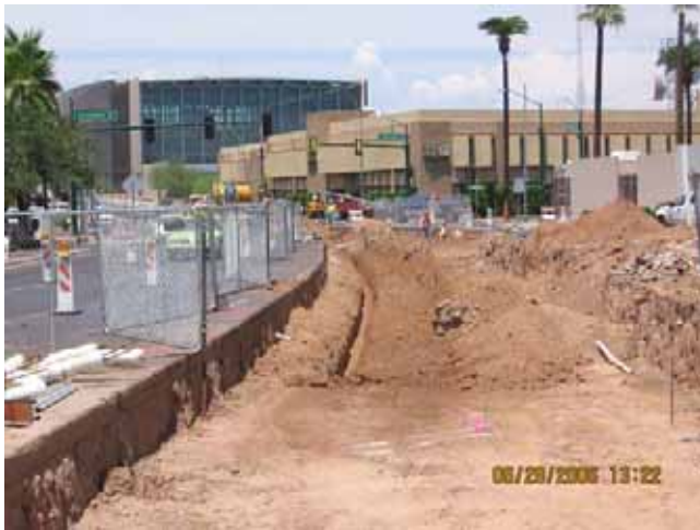
Excavation of 1 st Ave/Roosevelt Station Platform
