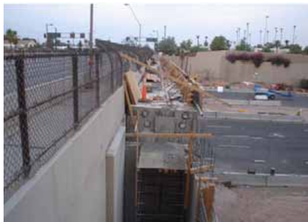
Pedestrian Bridges Lowered into Place at 101 Freeway
