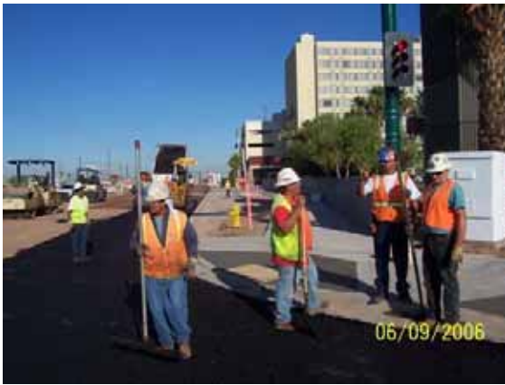
Paving 44 th and Washington Streets
