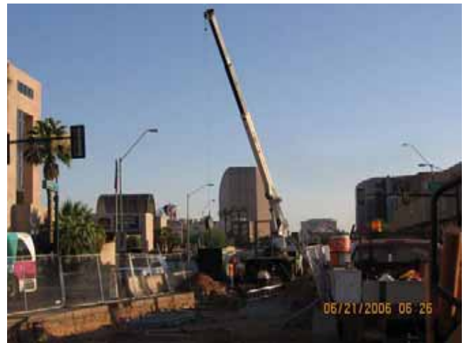
Setting Communication Manhole
