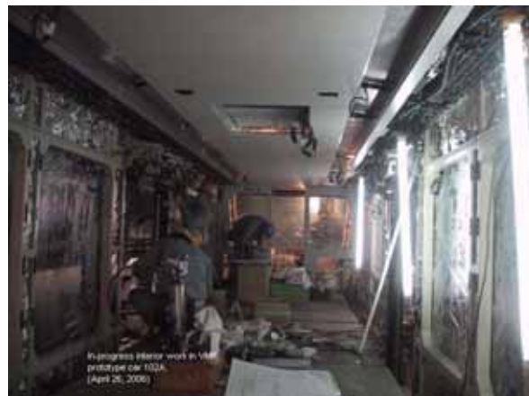
In progress interior work in METRO Prototype car 102.
