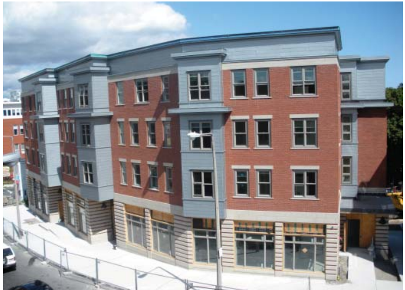
The Dudley Village project developed by the Dorchester Bay Economic Development Corporation in Boston will bring 50 affordable housing units to Roxbury.
