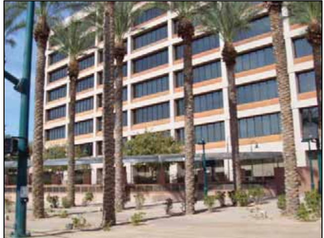
VIEW IS TOWARD THE NORTHWEST
