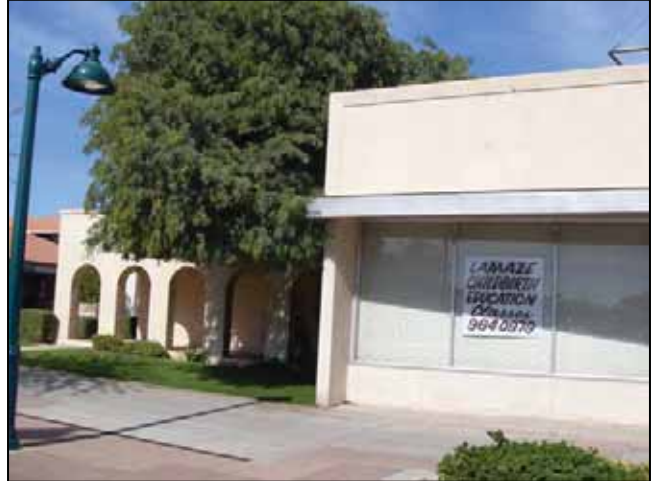
VIEW IS TOWARD THE NORTHWEST
