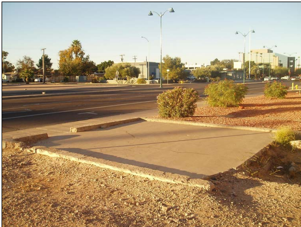
Figure 14. Commercial building foundation on north side of Main Street.
