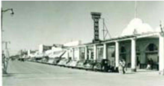
Figure 10 - Based upon the automobiles and the double acorn street lights at the Main Street median, this photo may date from the late 1940s. The Mission Revival Style building is the 1908 Chandler Court which is among the earliest reinforced concrete buildings in Arizona. (Mesa Southwest Museum)
