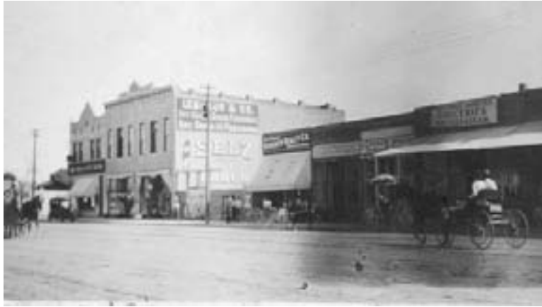
Figure 6 - Mesa's original town site had developed into a respectable central business district by the 1900s. Fired clay brick stores and businesses had replaced earlier vernacular adobe and wooden buildings. Main Street, flanked by boardwalks and concrete sidewalks, was not yet paved. Power poles along the front edges of the walkways soon would also support streetlights. (Mesa Southwest Museum 82-63.9)
