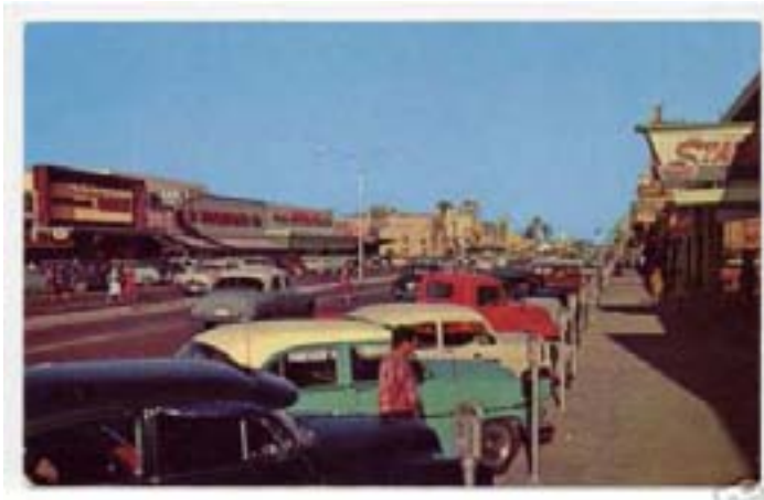
Figure 12 - During the late 1950s curbside parking meters appeared at the diagonal stalls to help manage the increasing parking problems in the post-World War II period. The centerline street lights were up-dated with taller standards with double cobra-head fixtures. (Mesa Southwest Museum)
