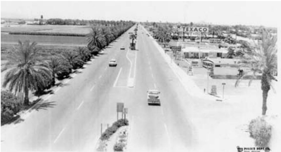
Figure 16 - In 1967 Mesa's Main Street west of Alma School Road was characterized by remnants of agricultural land (UA Extension Service Farm) and by low-density, automobile-influenced commercial development constructed during the Great Post-World War II Boom. (City of Mesa Police Department files)
