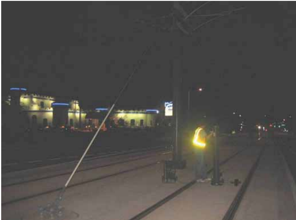
FIGURE C-2: IMPACT TESTING, EASTBOUND TRACK
