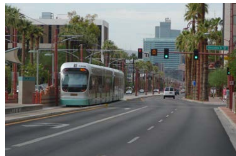
Example OCS with center poles between tracks
