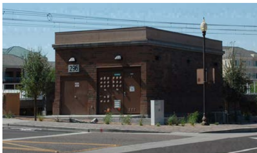
TPSS building at 3 rd St./Mill Ave. in Tempe
