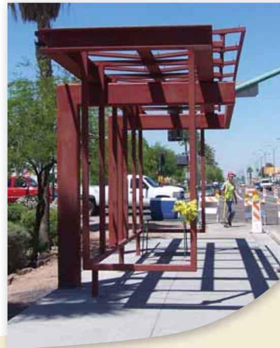
BRT station in Mesa under construction.
