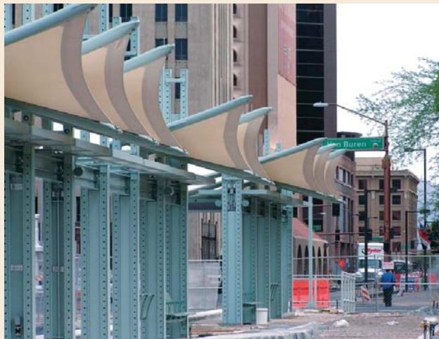
Light rail station features louvered shade canopies that will offer passengers shelter from sun and rain.
