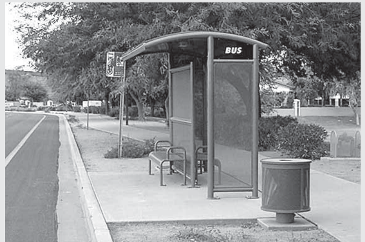
One of 86 bus shelters in the Town of Gilbert.
