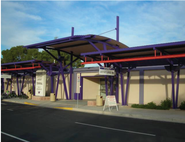
Entrance to Passenger Terminal
