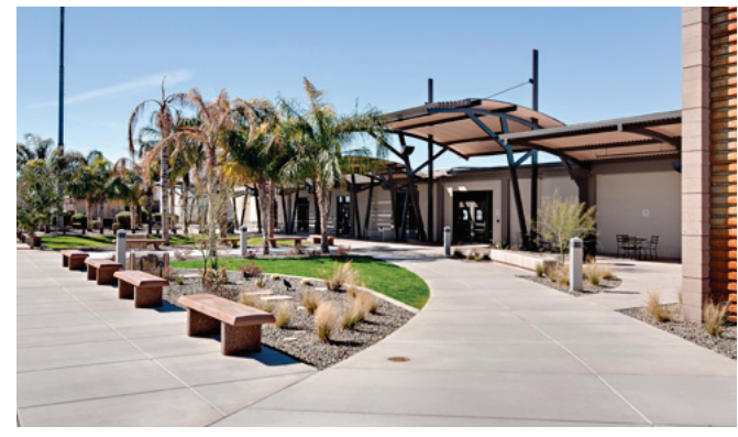
Passenger Terminal Courtyard (6033-2 S. Sossaman Rd.)
