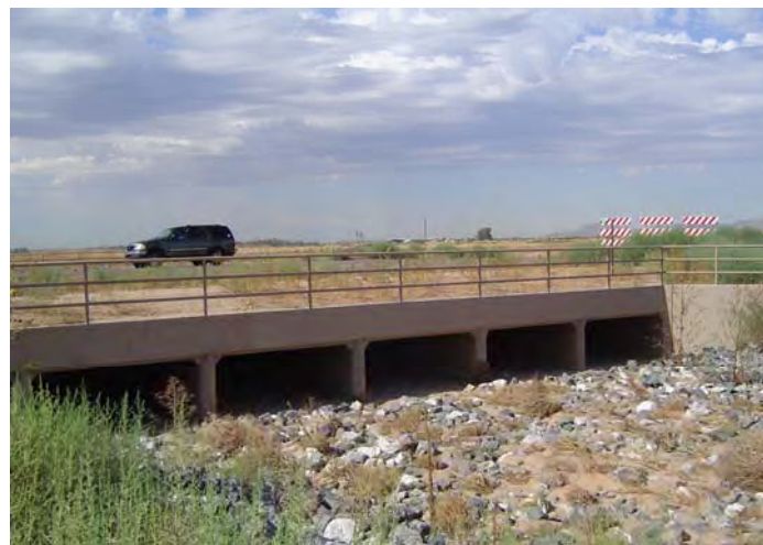
Existing Concrete Box Culvert West of Reems Road
