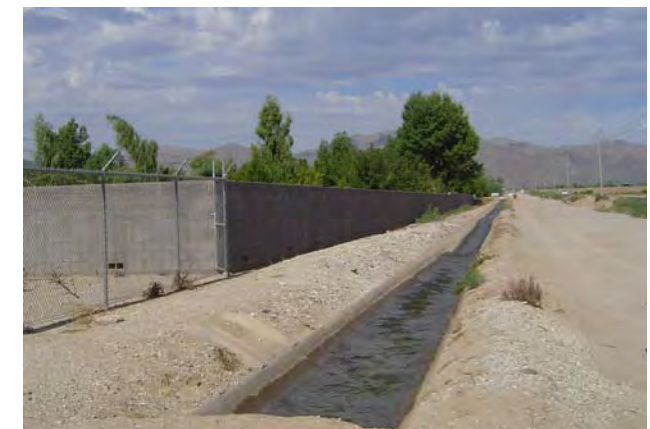
Existing MWD Lateral 8
