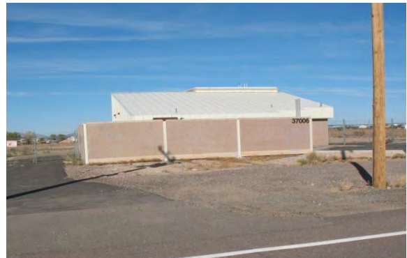
CenturyLink telecommunications facility
