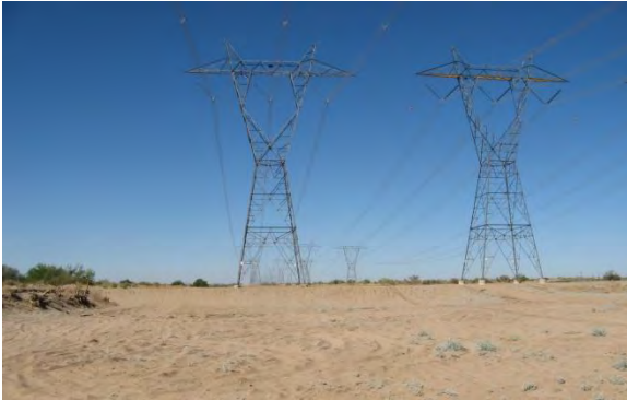
Existing 500kV transmission lines
