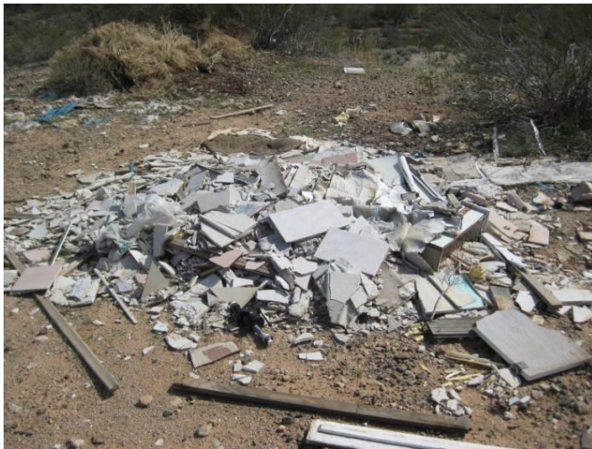
Photograph 5. Illegal dump site with construction debris
