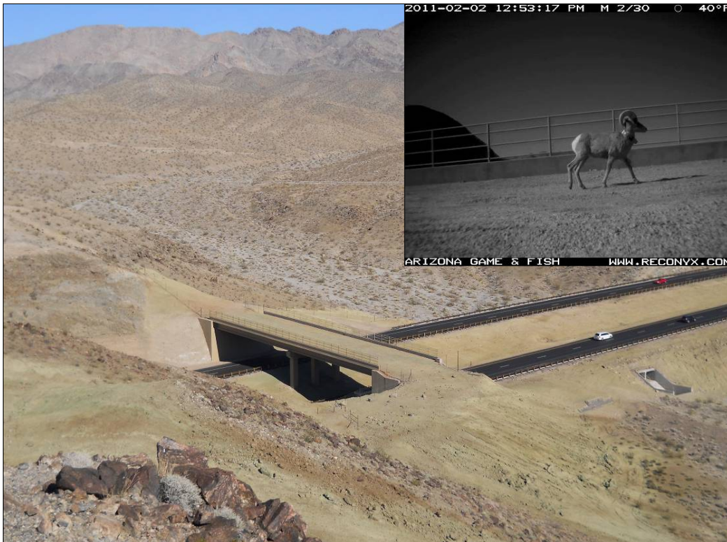
Figure 26. Completed U.S. 93 Wildlife Overpass at Milepost 5.1 (looking east). Inset Photograph Shows One of the First Desert Bighorn Sheep Highway Crossings via the Overpass.
