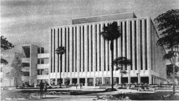
Addition to Life Sciences Building
