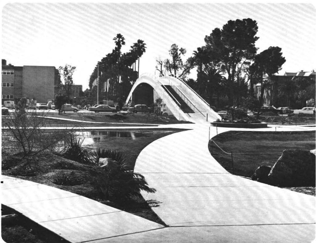
Palo Verde Halls pedestrian bridge crosses University Drive.
