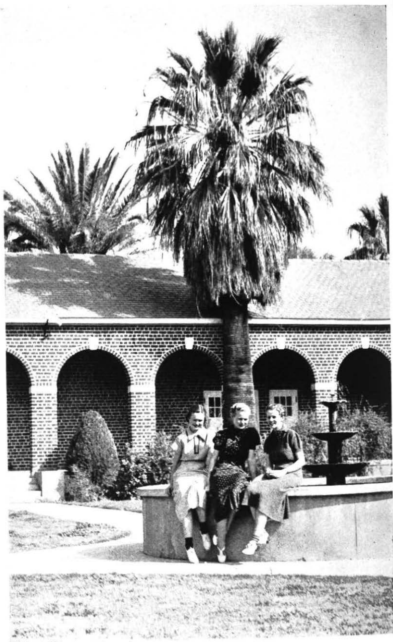
THE FOUNTAIN, PATIO OF CAMPUS TRAINING SCHOOL
