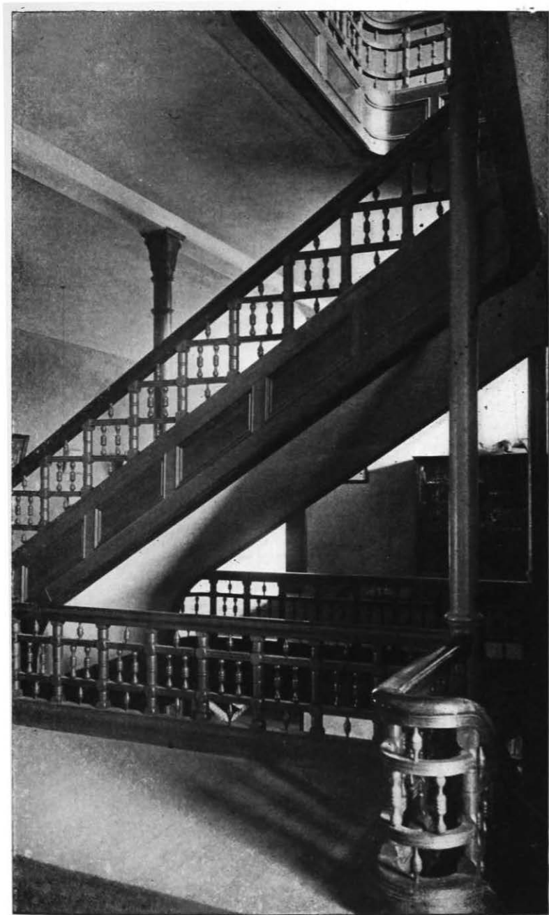
STAIRWAY IN MAIN BUILDING
