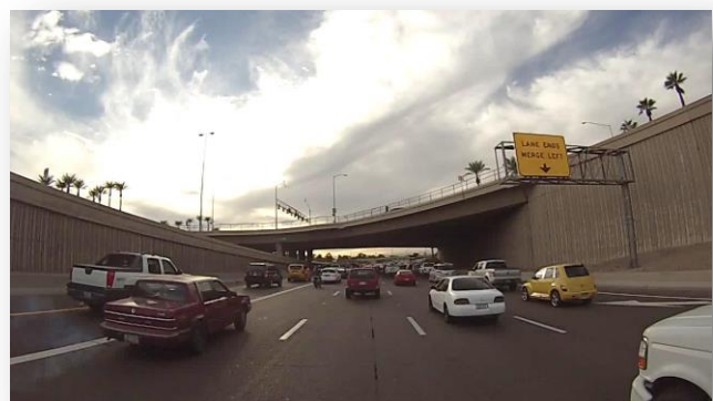
Figure 19. Westbound Lane Drop West of 7th Ave Exit; Note queuing in right two lanes
