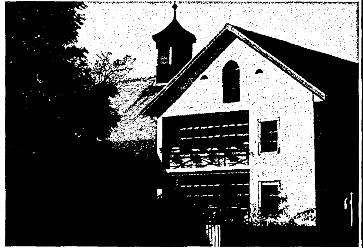
▲ The Thunderbird facility in Archamps, France is located in the International Business Park close to the Swiss/French border near Geneva.
