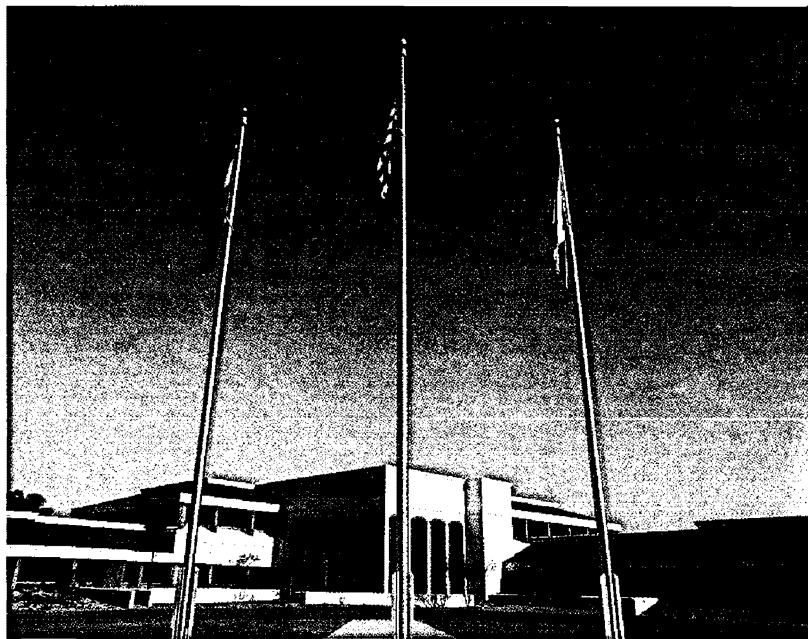
The new World Business/Administration Building houses most of the administrative offices in its Joan and David Lincoln Administration Wing. Offices located there include Admissions, Housing, Financial Aid, Student Affairs, Academic Affairs, Business Affairs, Personnel, Alumni Relations, External Affairs, and the President's Office.
