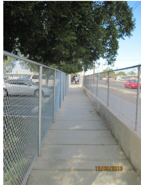
Pedestrian access way leading to pedestrian gate at the intersection of 12th Street and Avenue A
