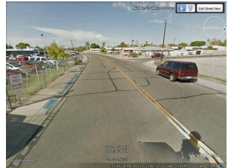
Blue painted curbing on Palmcroft Drive west of school exit drive
