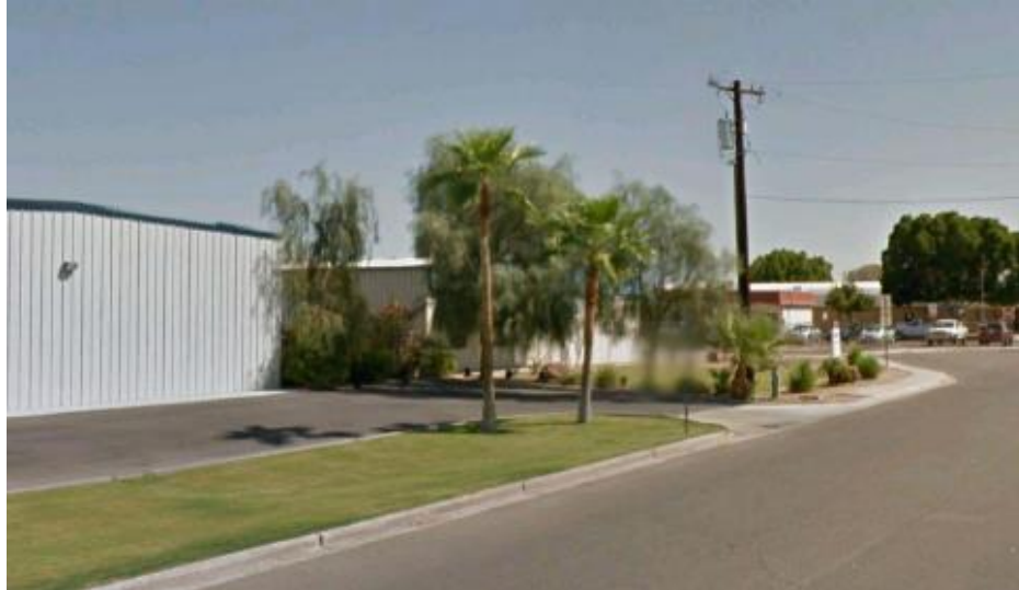
Sidewalk gap on north side of 22nd Street
