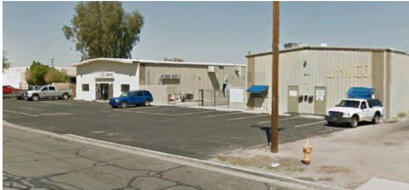
Industrial land uses north of school
