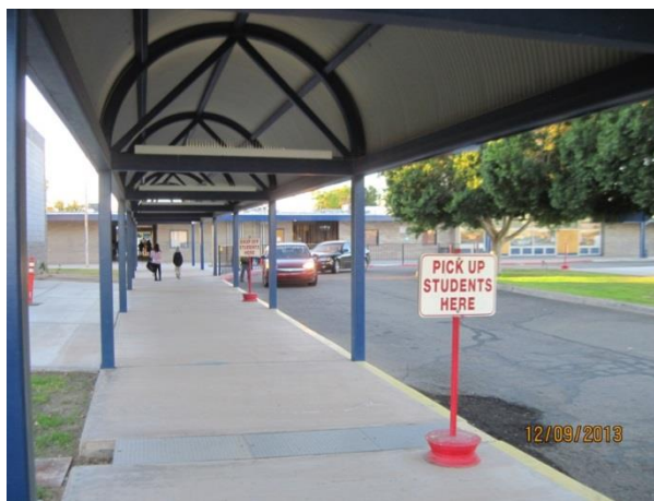
Morning Drop Off at family vehicle loading zone
