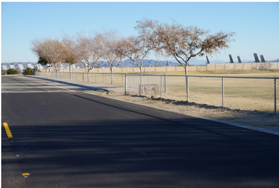
Sidewalk truncates on the east side of the roadway, north of Otondo Elementary
