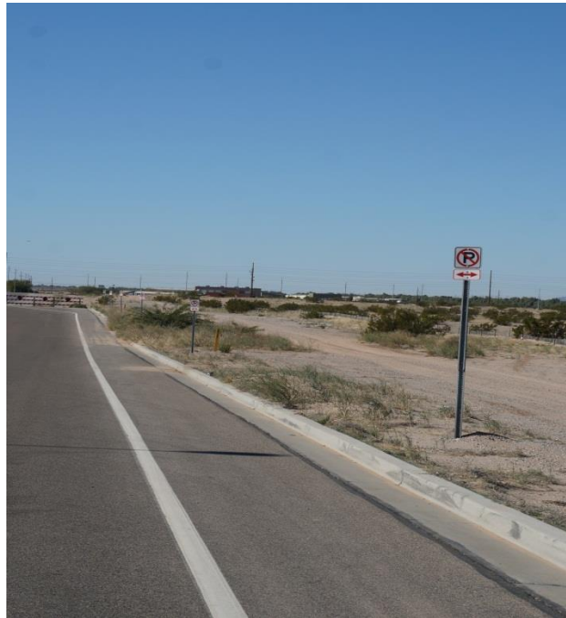
No Parking signs along the north side of 28th Street
