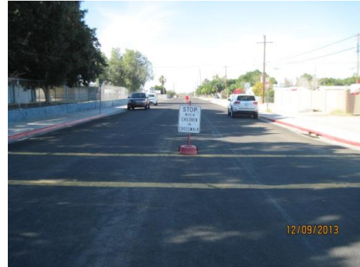
Mid-block crosswalk in front of school
