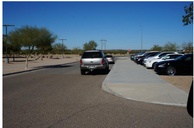
Unauthorized overflow parking along egress driveway
